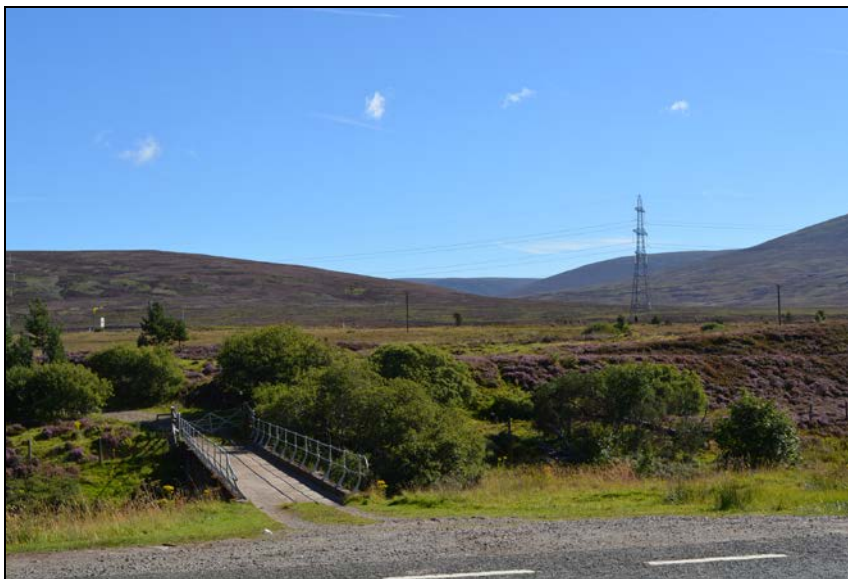
Photograph 14-1: Existing SSE Aqueduct track and view of the proposed A889 tie-in location
