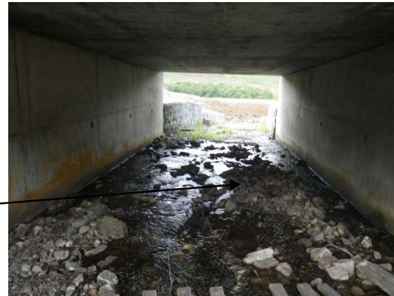
Photograph 11.4.3.115- Downstream under crossing
