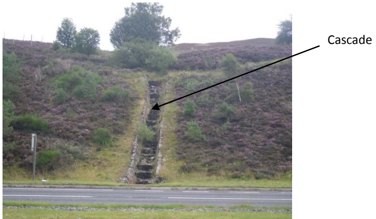
Photograph 11.4.3.124- Cascade upstream of crossing
