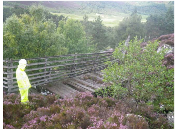
Photograph 11.4.3.143 - Bridge crossing channel
