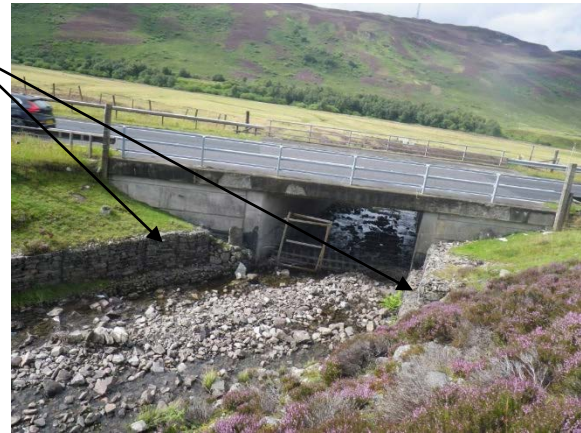
Photograph 11.4.3.117 – Downstream to crossing
