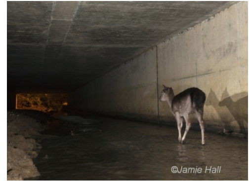
Photo 2 Fallow deer crossing box culvert underpass beneath 6-lane M25 Essex
