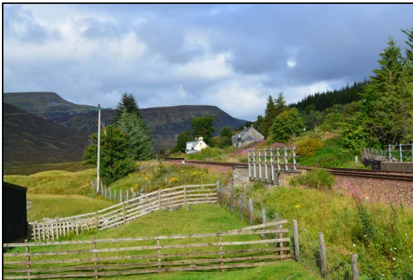
Photograph 8-1: Photograph of Station House and Station Cottages
