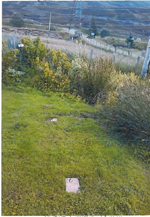
**Photograph 1:** Septic tank inspection holes
