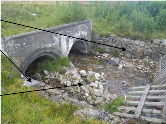
11.4.3.100 - Deposition of coarse material in culvert entrance
