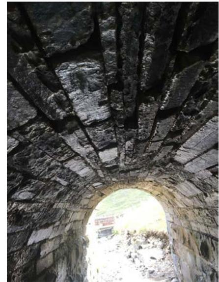
Photograph 3-9: Gaps between mortar in stonework
