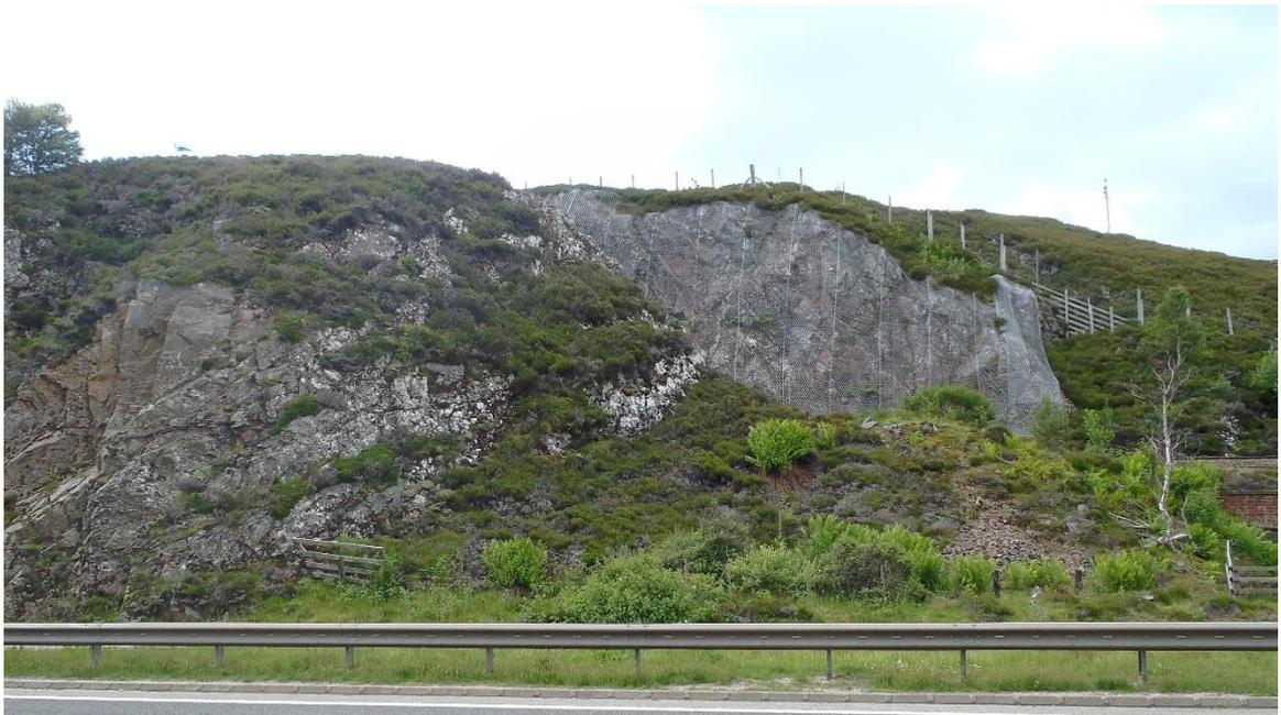
**Photograph 4.3: Photo at Slochd showing how poorly designed seams can create a 'striped' effect**
