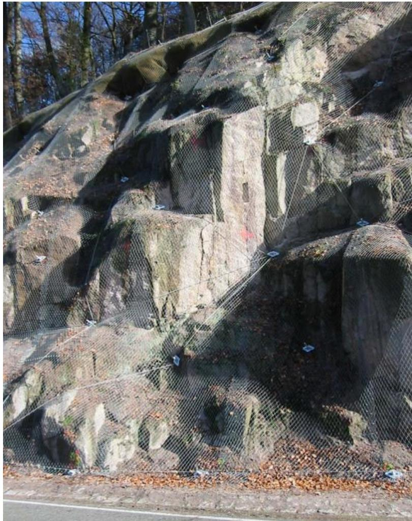
Photograph 4.1: Photo showing how contouring mesh can reduce its prominence (Image Credit: Geobruigg)
