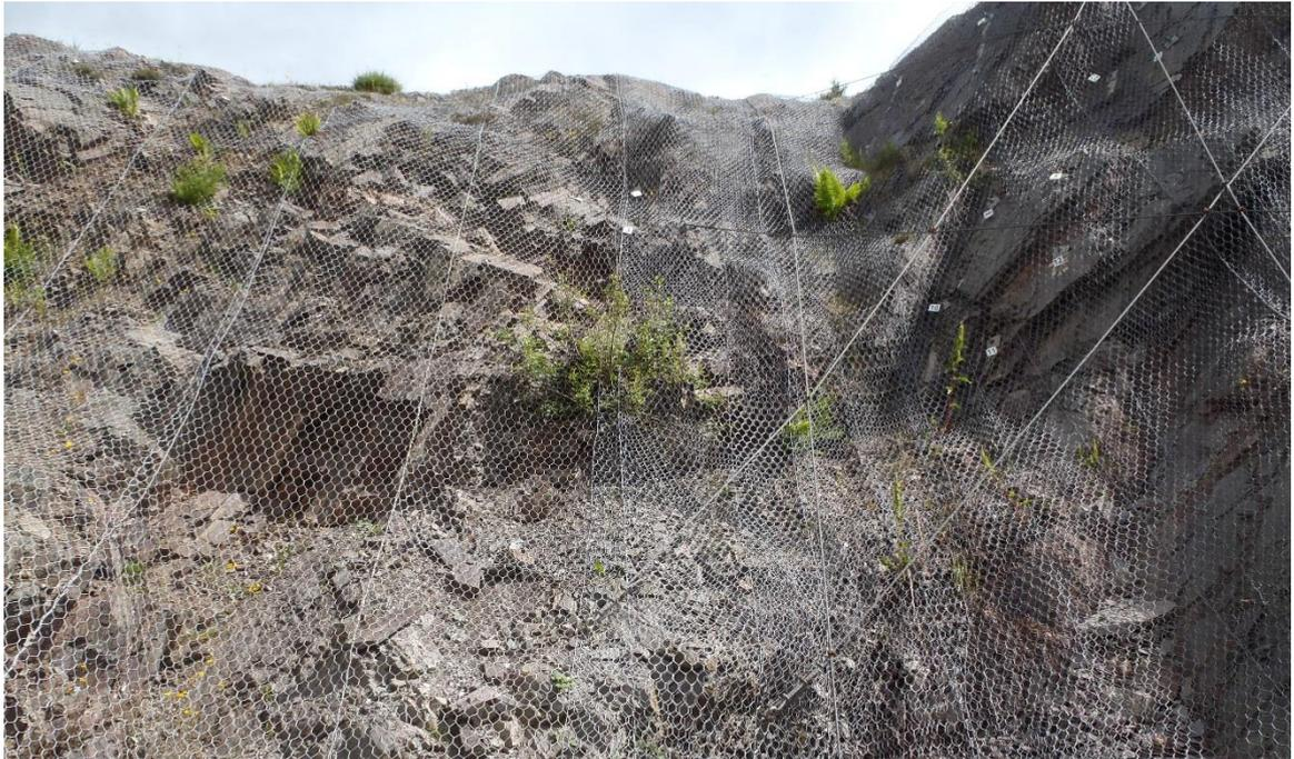
**Photograph 4.2: Photo at Slochd showing how cabling can detract from views of the rock face**
