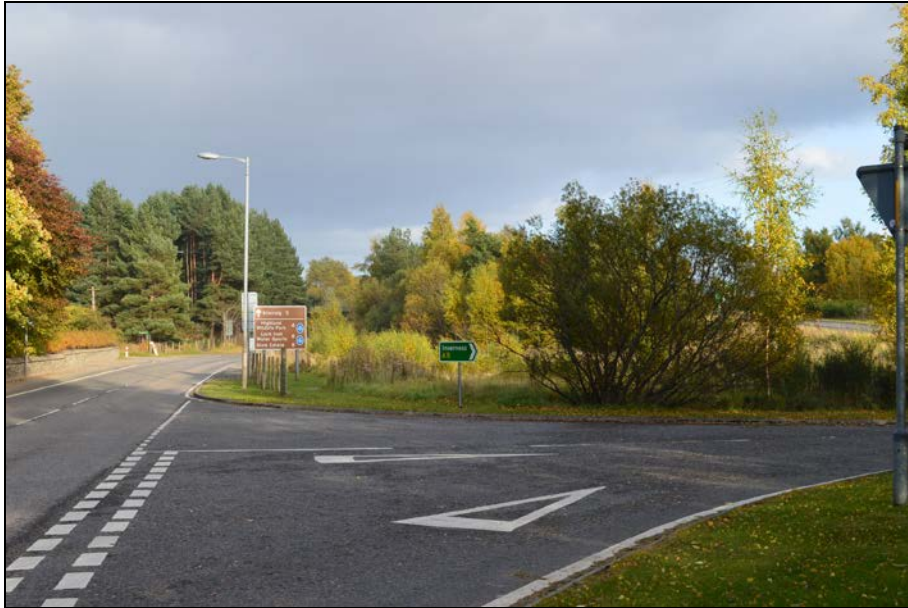
Photograph 9-11: A86/A9 slip road junction at Kingussie, providing access to and from the northbound carriageway of the A9
