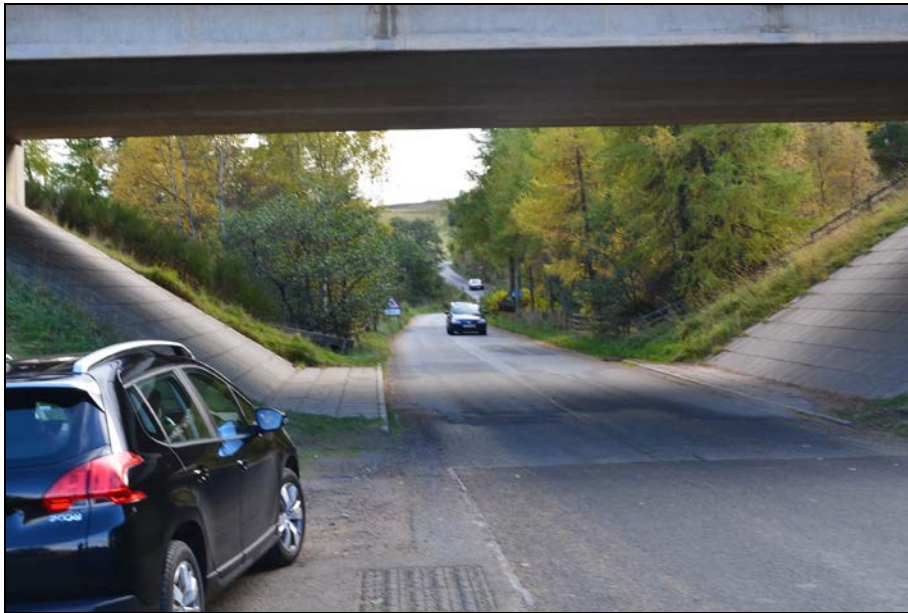
Photograph 9-10: NCN7 and East Highland Way, on-road section from Kingussie
