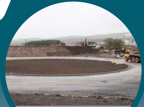
Progress at Highfield roundabout
