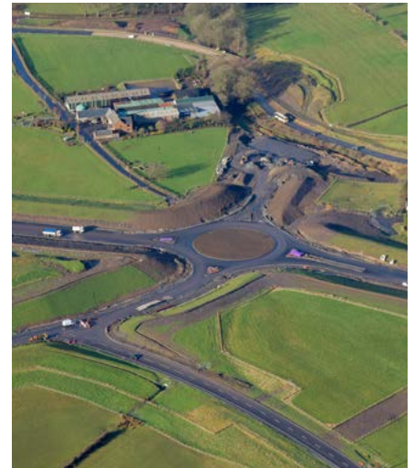
Aerial photo of Highfield Interchange
