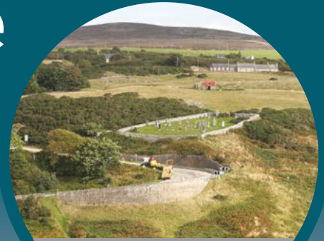
Existing road at Berriedale Braes
