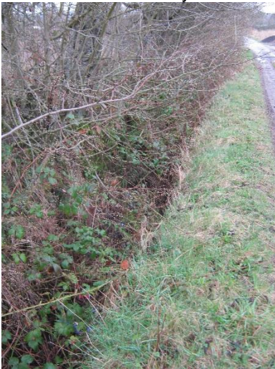
Photograph 9: Roadside channel (NH 69943 45681)
