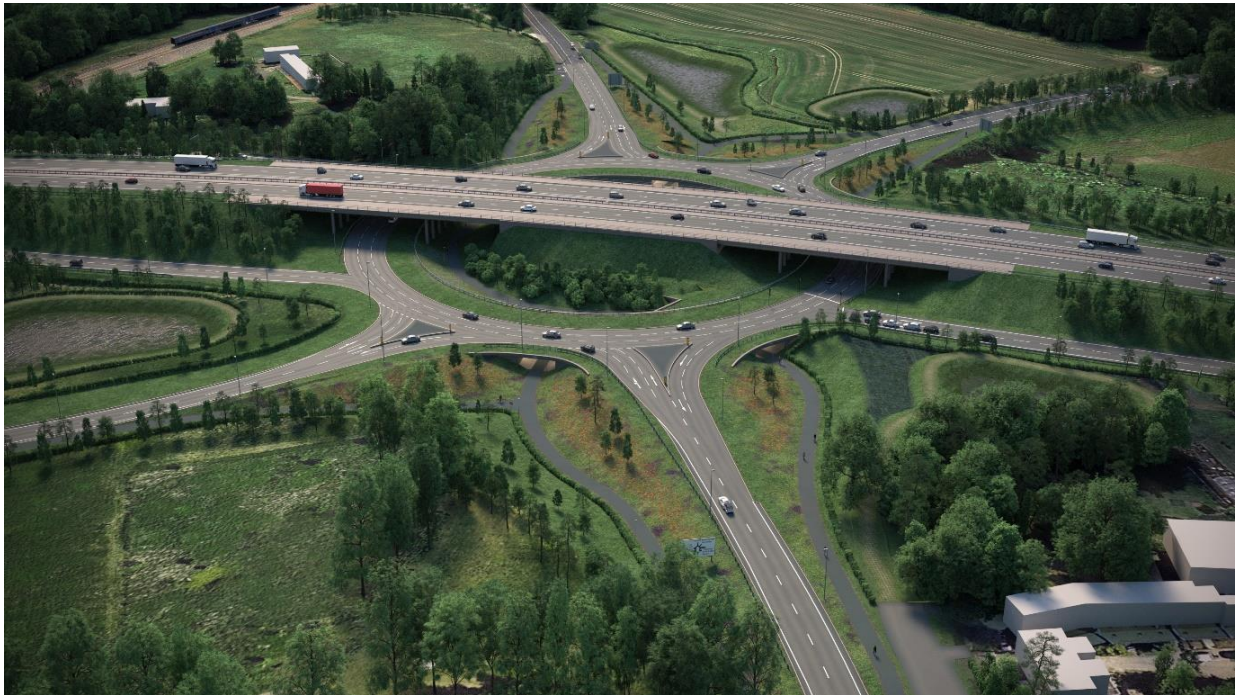
Plate 5-4 View of the Proposed Scheme looking South along the A7 North towards Dalkeith
