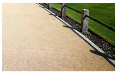
Fig. 36 Exposed aggregated concrete with low kerb edge, Leicester Public Real (AECOM)
