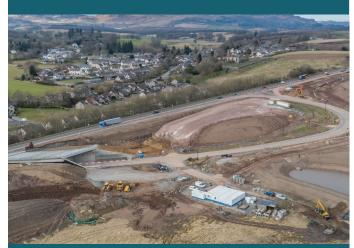
The beam lift operation, which included 23 pre-cast concrete beams, was completed during overnight closures in March 2020 following several weeks of backfill operations
