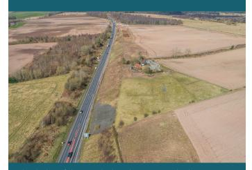
The design of the new dual carriageway required a substantial volume of earth to be removed at this location to accommodate the new A9 southbound
