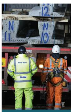
Precast bridge beams being delivered to site ahead of the nightshift to install them
