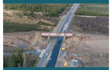
Nine pre-cast concrete beams weighing a total of 390 tonnes were installed during overnight closures of the A9 to create 'The Green Bridge'
