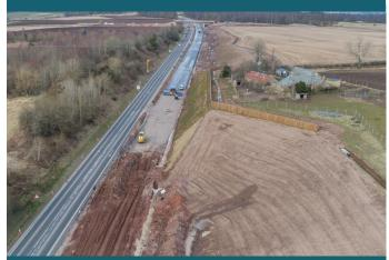
The new line of A9 southbound carriageway takes shape following completion of the soil nail wall to retain the embankment, protecting the neighbouring property
