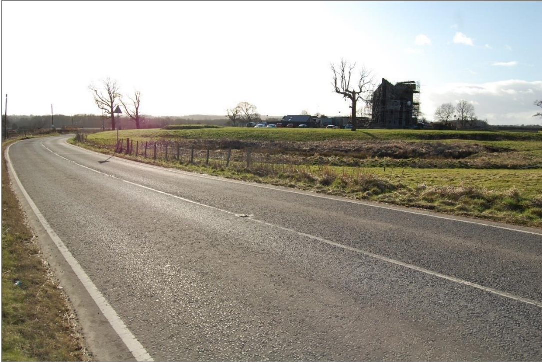
PLATE 5.3: VIEW OF DUNTARVIE CASTLE FROM NORTH APPROACH ALONG B8020 AT JUNCTION WITH BULLYEON ROAD
