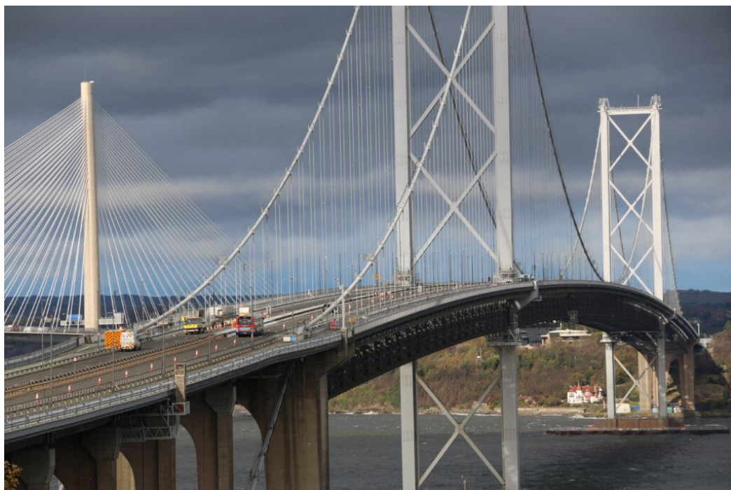
Figure 2. The Forth Road Bridge. Source: New Civil Engineer.
