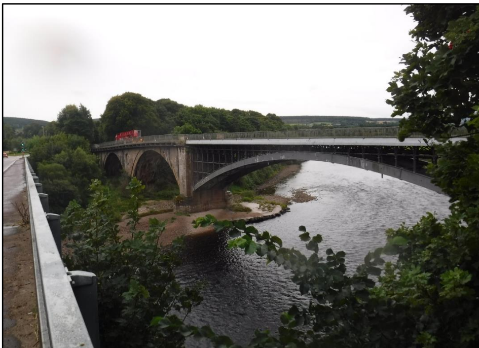
Figure 2. The A96 409 Fochabers Old bridge (looking south). Source: BEAR Scotland.
