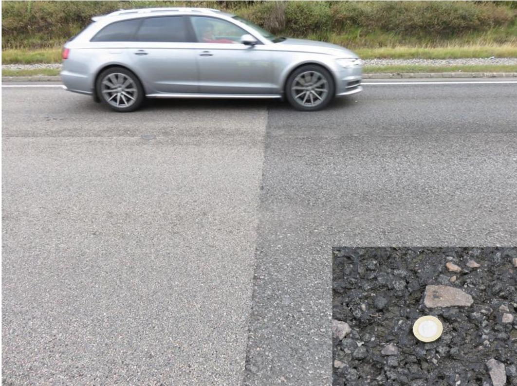
**Figure 3.5: Aggregate loss at IP43 - material (including close-up) on the right**
