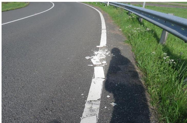
**Figure 4.11: Failed road marking**
