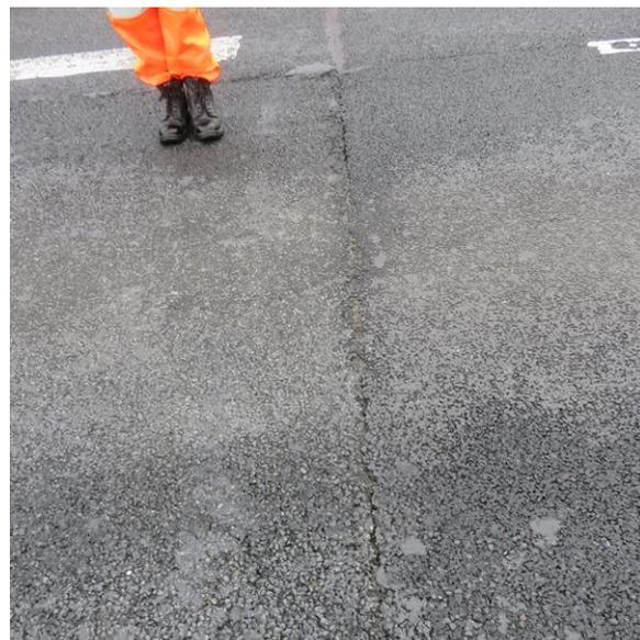
**Figure 3.6: Open joint at IP16**
