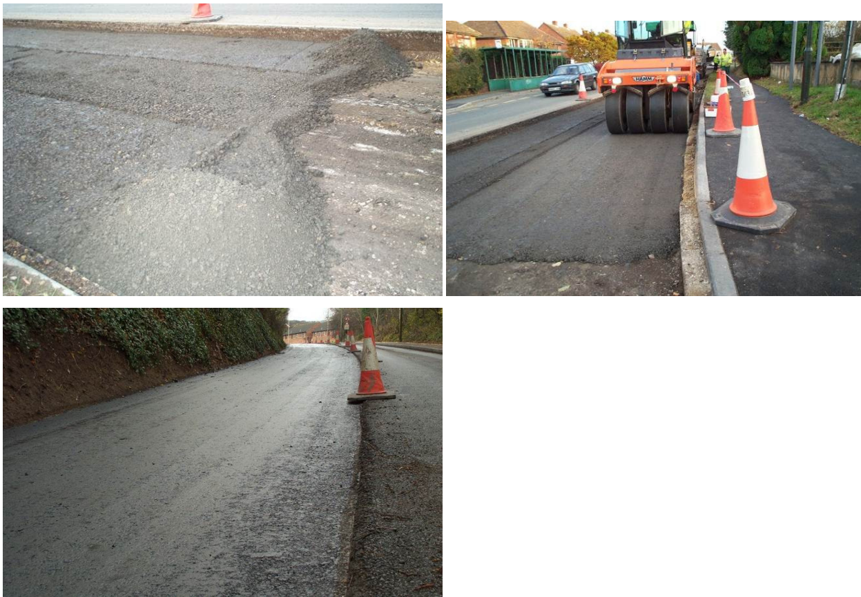
Figure 3: Spreading/laying, compaction, bond coating of VE CRBM
