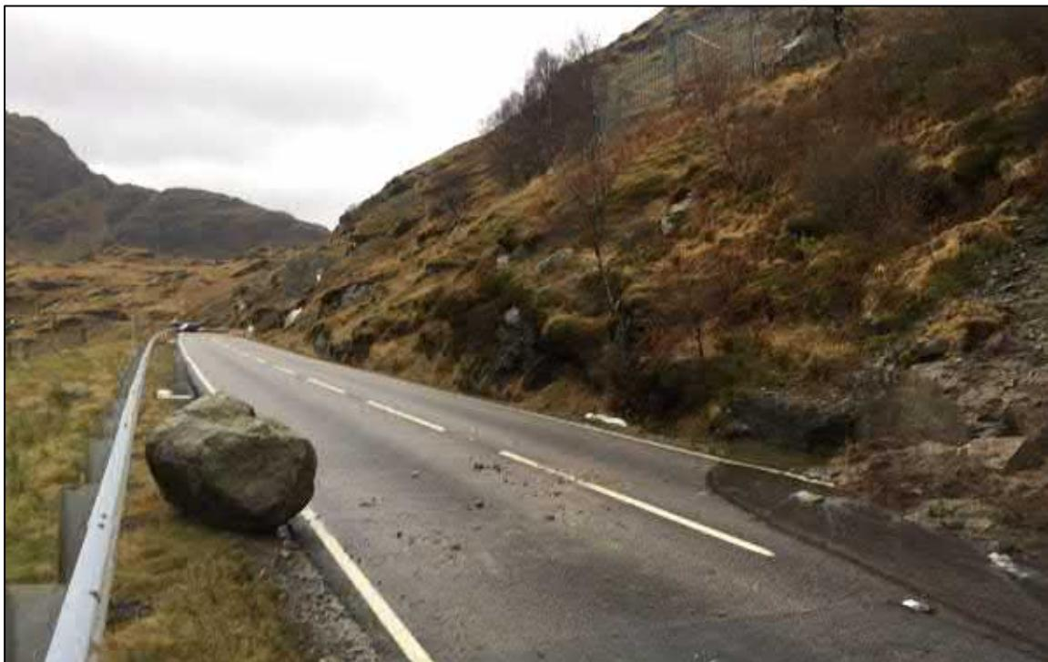
Photograph A-3: Photograph of the boulder that impacted the A83 on 30<sup>th</sup> December 2015 as a result of soil movement on the slope below the Phase 8 debris barrier.
