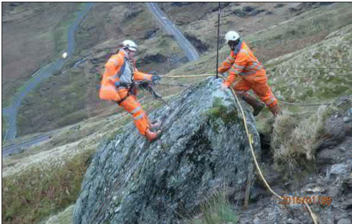
Photograph A-5: Photograph of potentially unstable boulder identified following the December 2015 debris flow being drilled so that it can be broken up using explosives.
