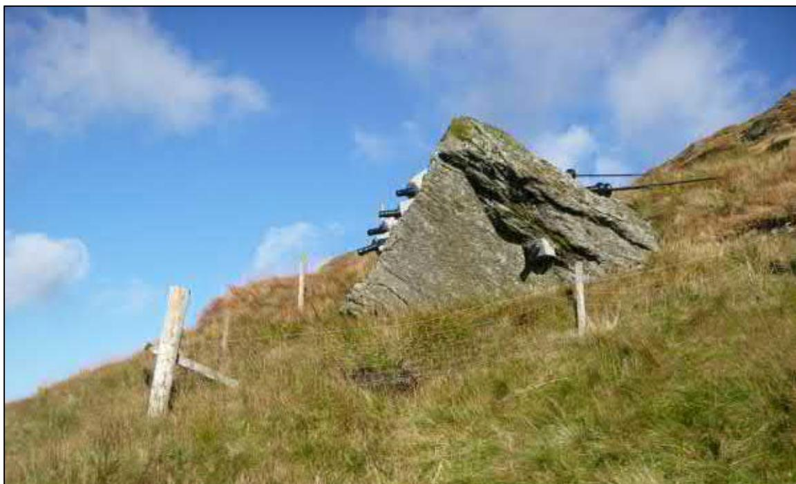
Photograph A-6: Photograph of a potentially unstable boulder following installation of a restraining system in 2015.
