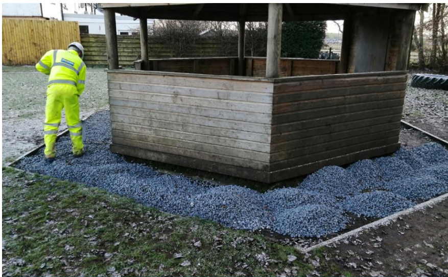
Levelling off gravel around the outdoor classroom
