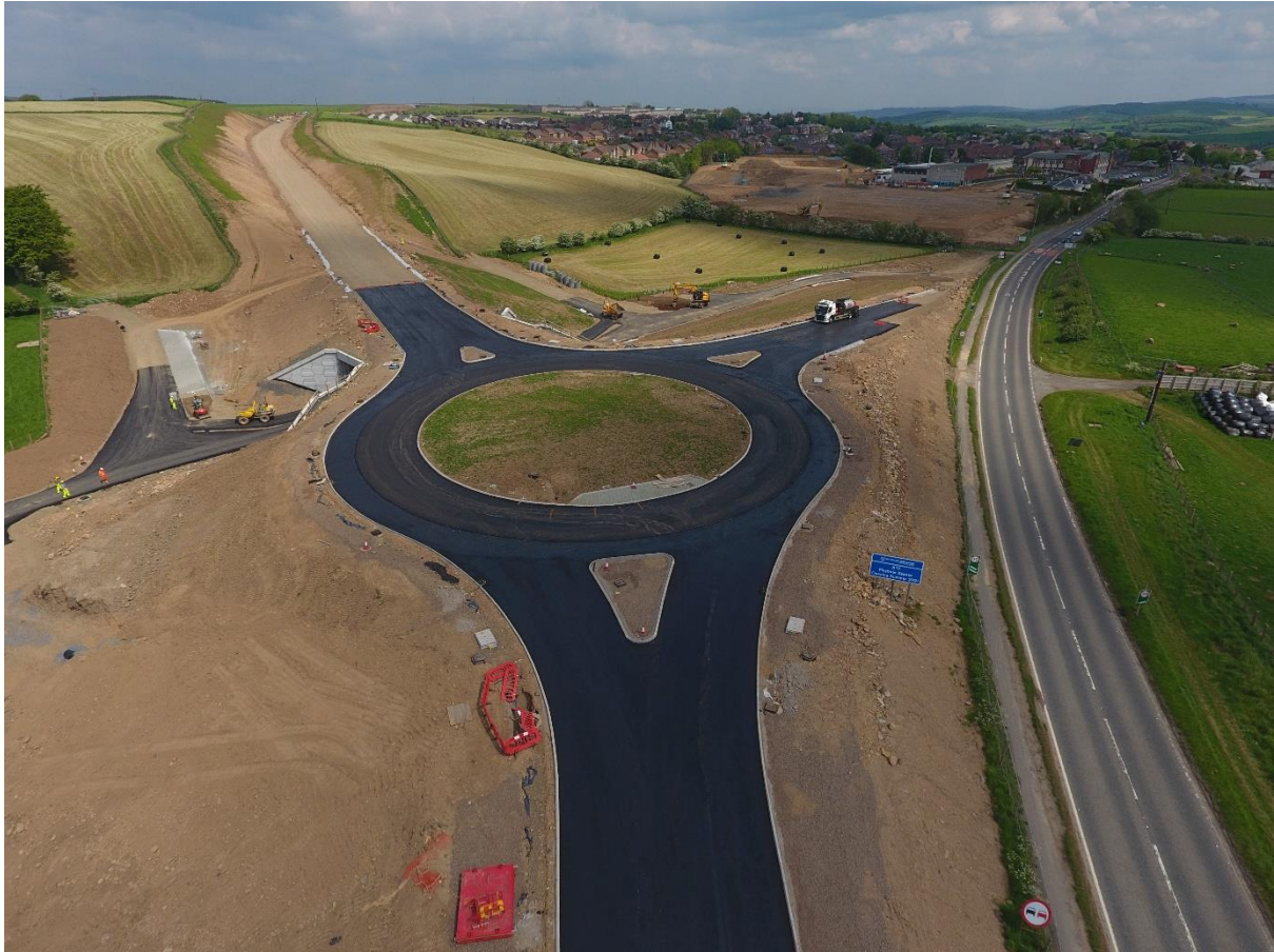
Construction of the new roundabout at Broomknowes
