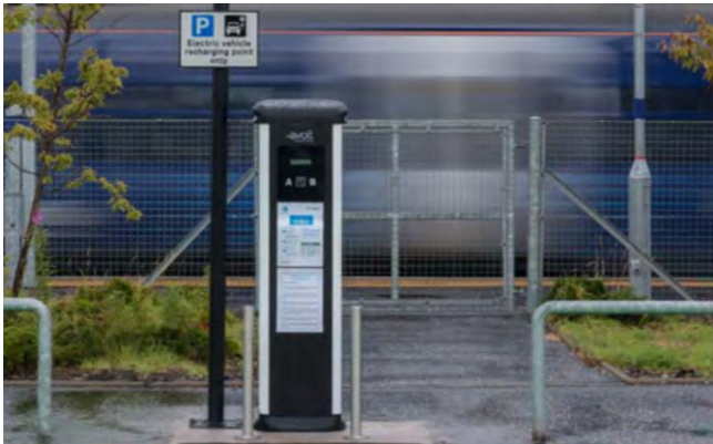
One of the new electric vehicle charging points
