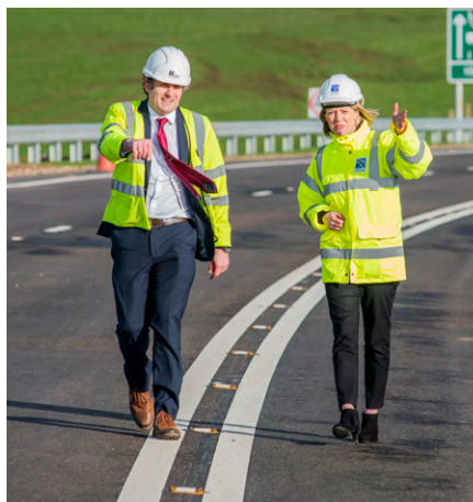
Minister for Transport, Jenny Gilruth, hears from Jonathan Wills, Wills Bros, about the construction of the Bypass.
