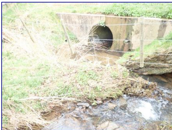
Figure 2 - A68 240 C35 New Blainslie culvert. Source: BEAR Scotland
