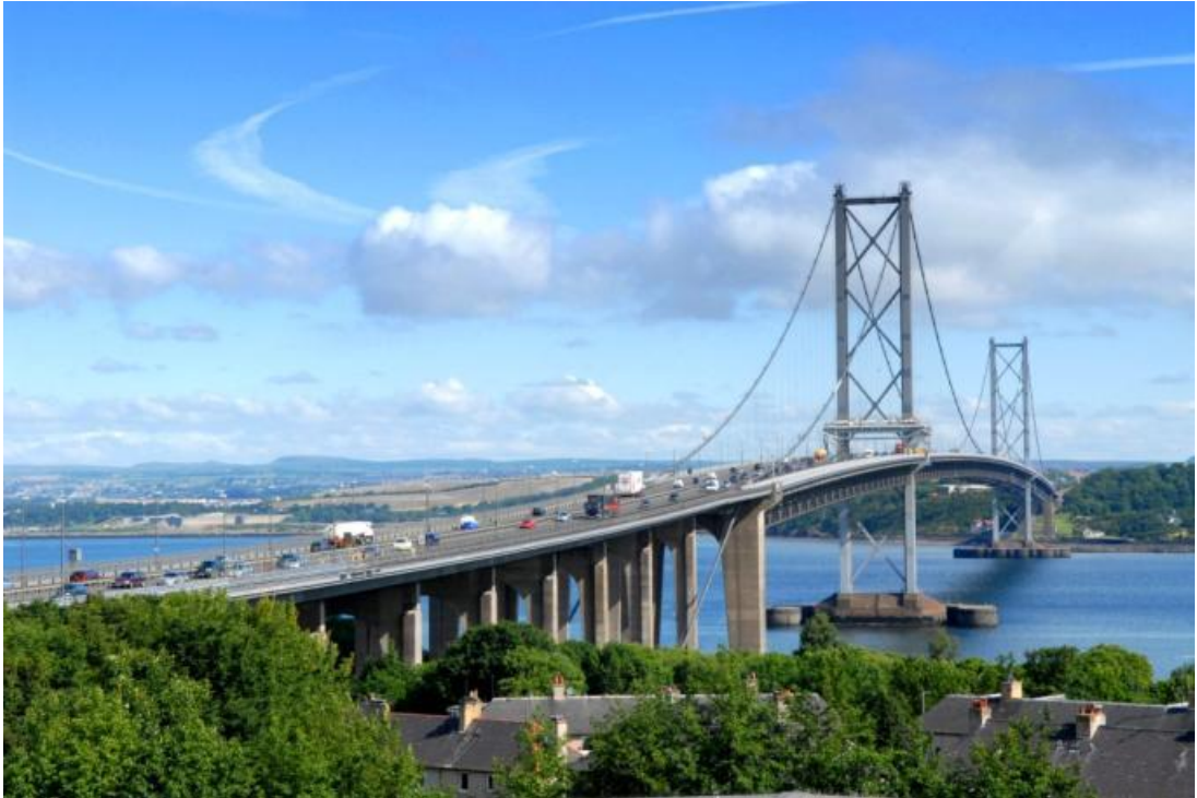
Figure 4.15.16.A – Forth Road Bridge
