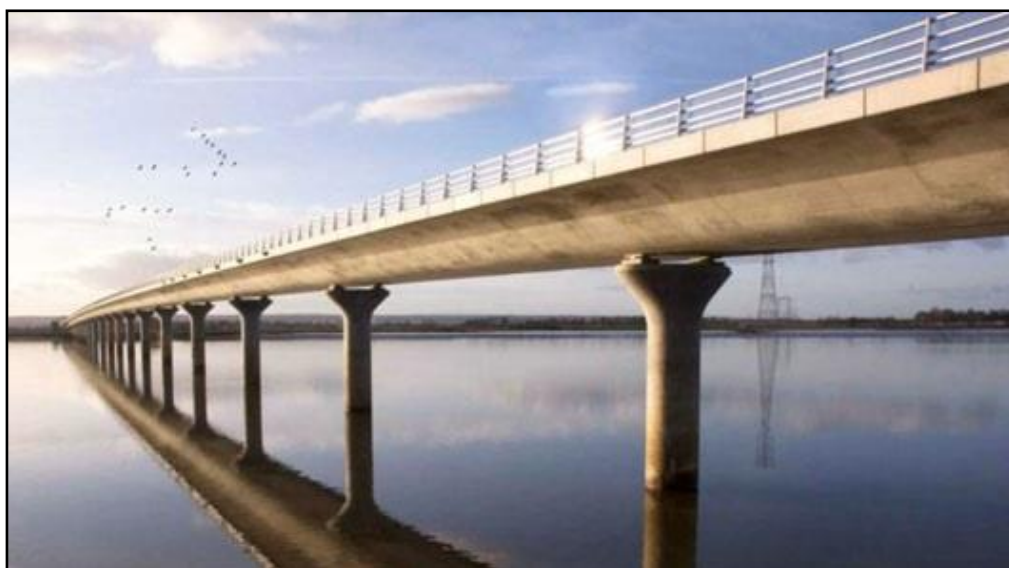
Figure 4.15.8.A - A876 50 Clackmannanshire Bridge
