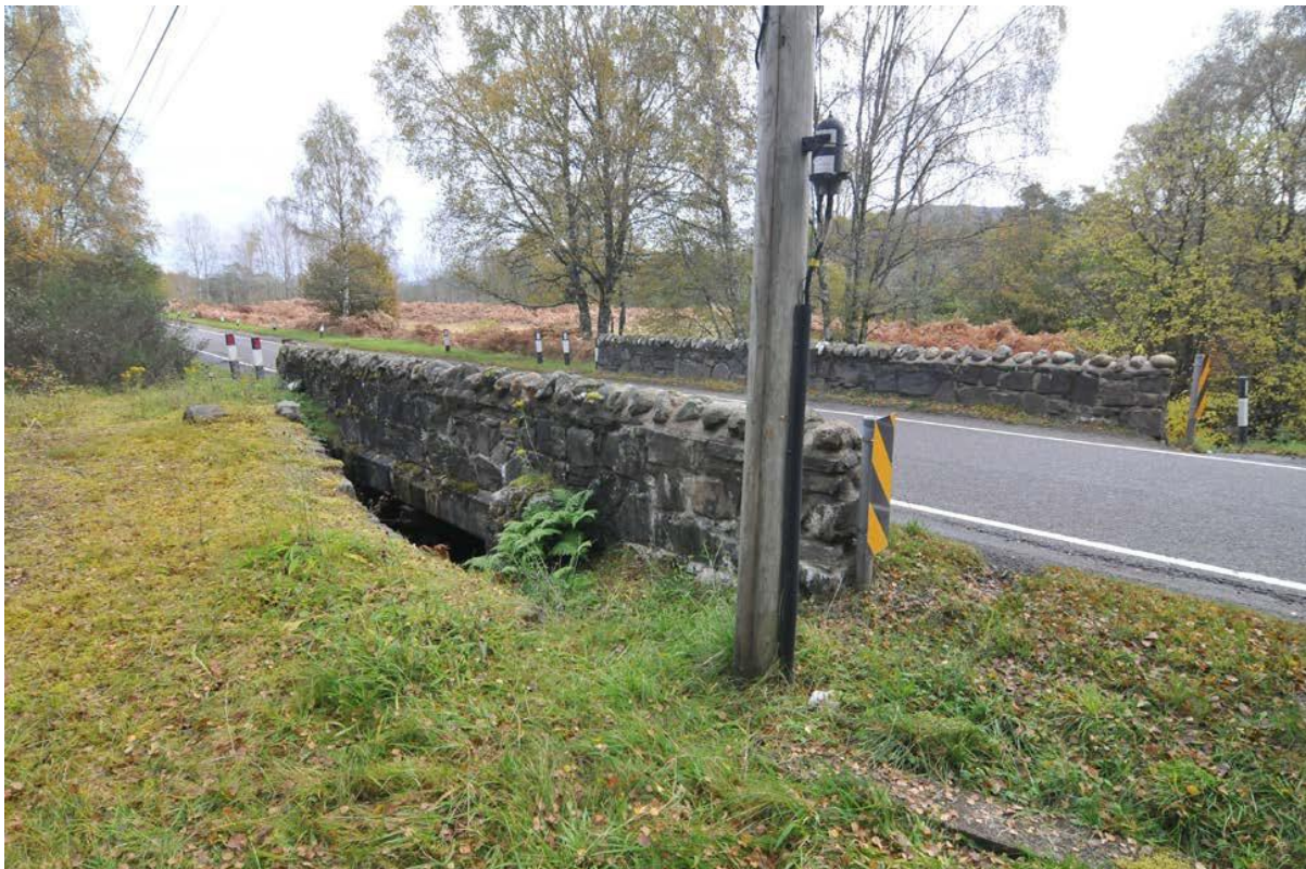
Figure 8 - New Bridge, oblique view of north-facing elevation
