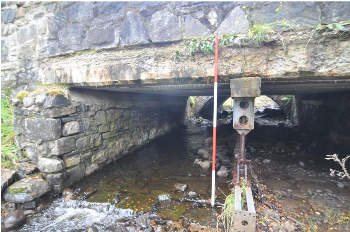
Figure 10 - New Bridge, below deck detail showing overflow race
