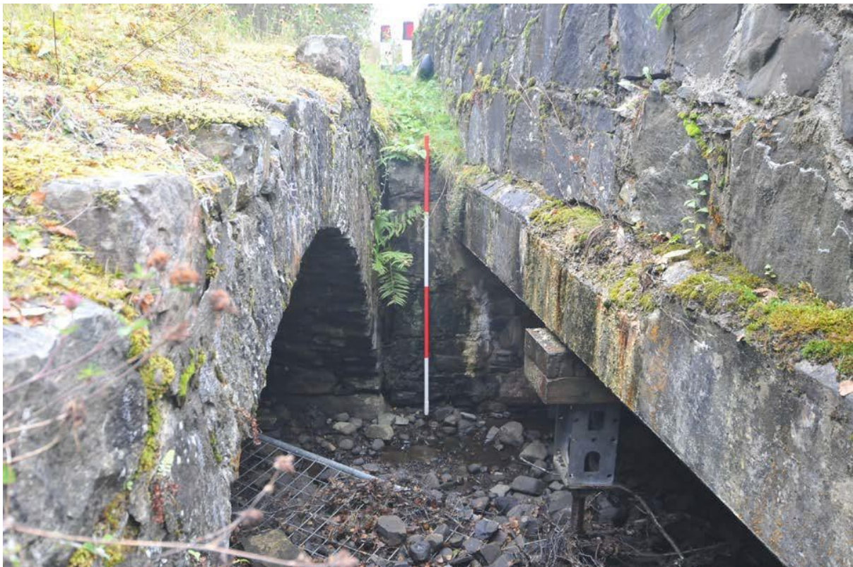
Figure 14 - Old bridge, oblique view of south-facing elevation and gap between bridges
