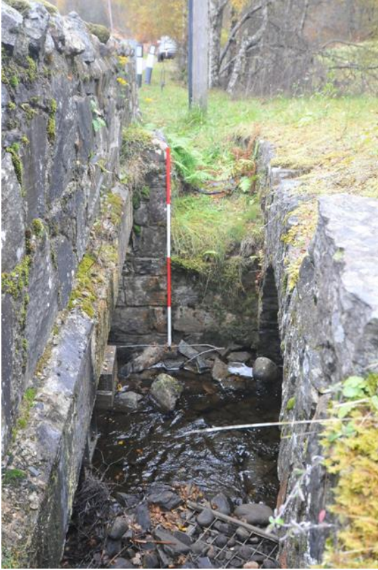
Figure 15 - Old bridge, detail of gap between the bridges
