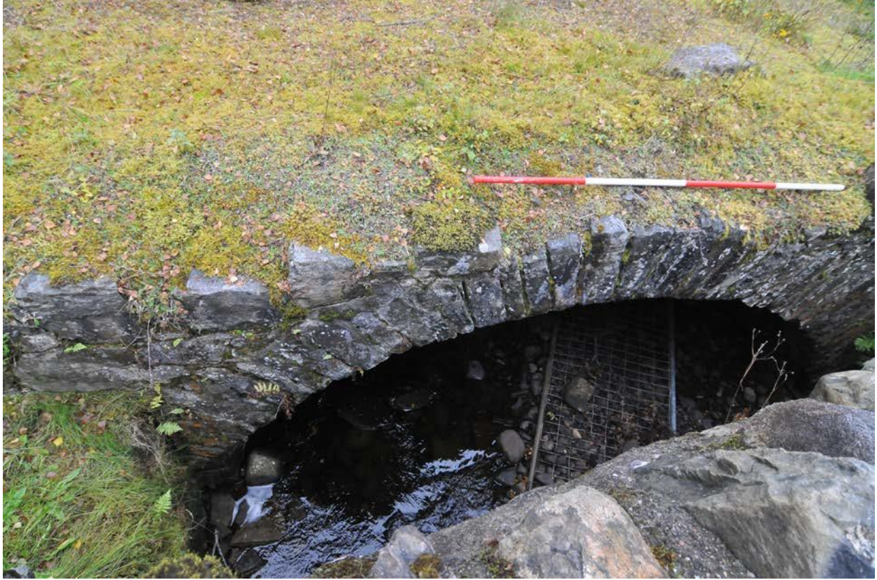
Figure 13 - Old bridge, oblique view of south-facing elevation
