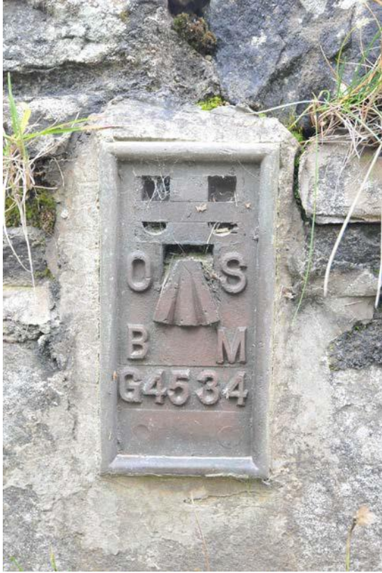
Figure 11 - New Bridge, north parapet, flush bracket detail
