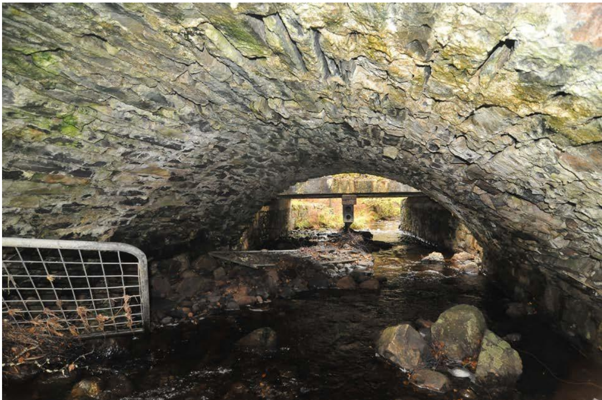
Figure 16 - Old bridge, detail of segmental arch
