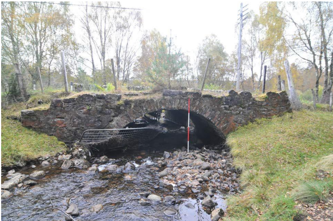
Figure 12 - Old Bridge, north-facing elevation
