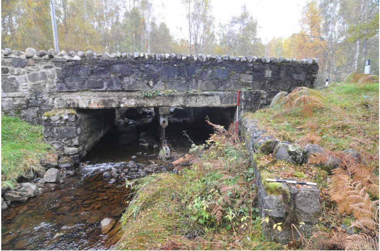
Figure 9 - New Bridge, south-facing elevation
