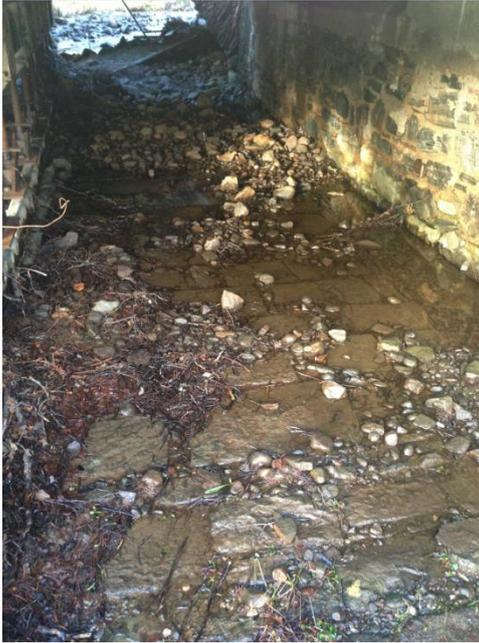
**Figure 2.3 View of invert showing brick laid stone arrangement**
