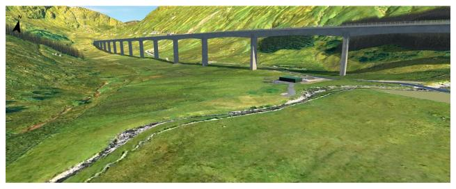
Figure 5-34 - Visualisation of the Purple Option Post Tensioned Concrete Balanced Cantilever Viaduct looking north up Glen Croe
