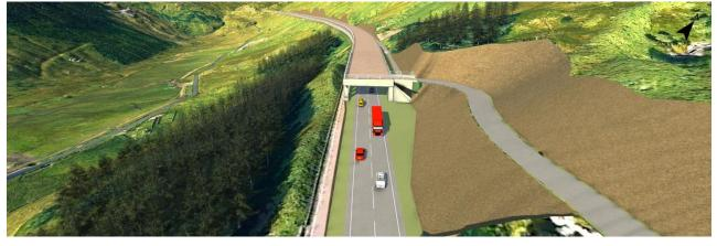
Figure 5-14 - Visualisation of the Brown Option Debris Flow Shelter looking north up Glen Croe from Croe Water
