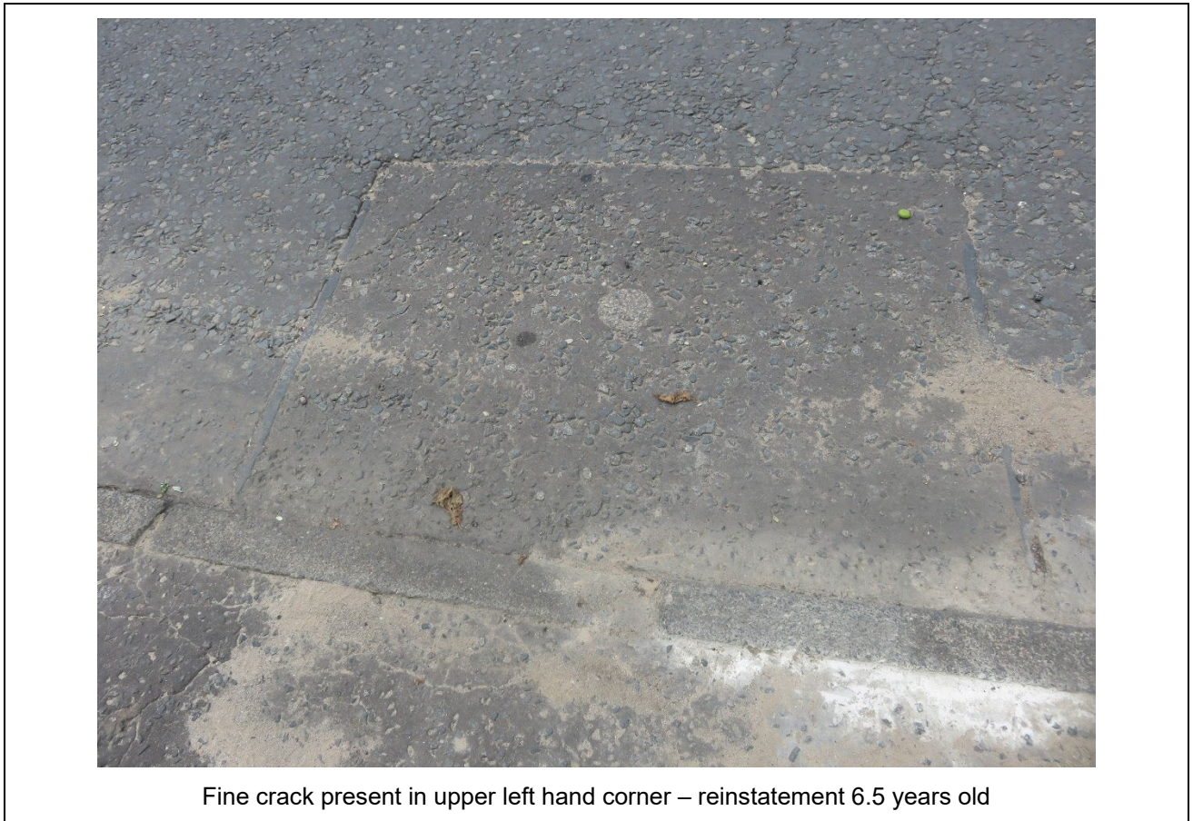
Figure 5-4 - Acceptable cracking
