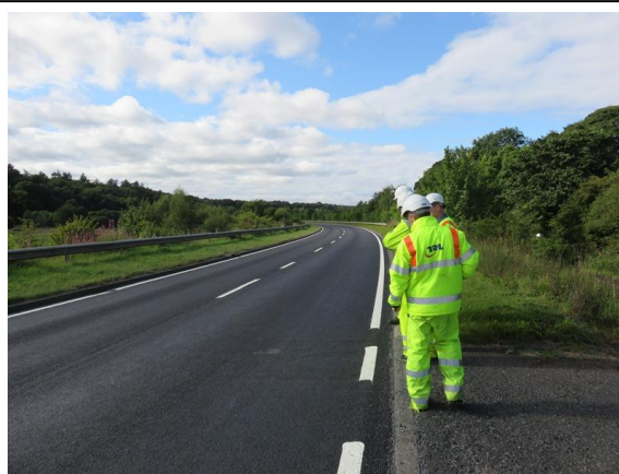
Figure 4.9 Treated surface dressing
