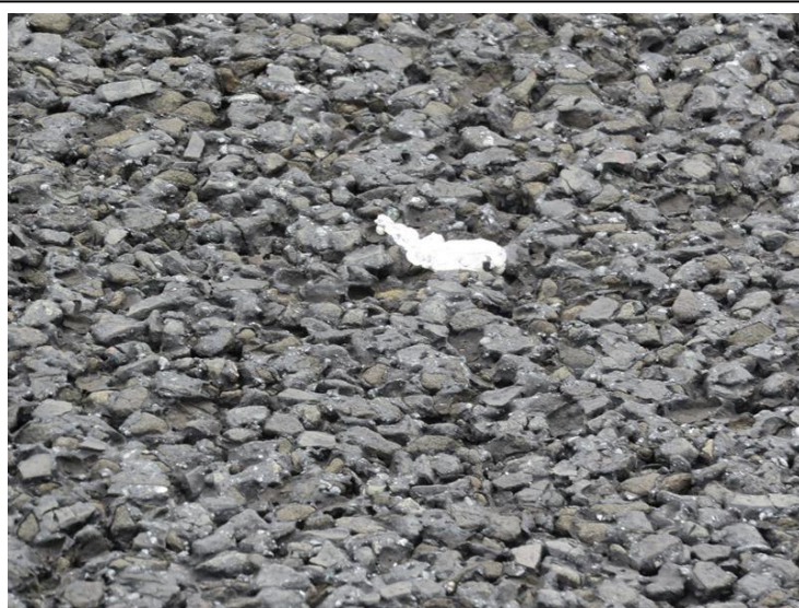
Figure 3.4 Aggregate loss at IP4
