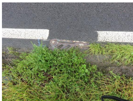
Figure 4.7 Choked gully (IP30)
