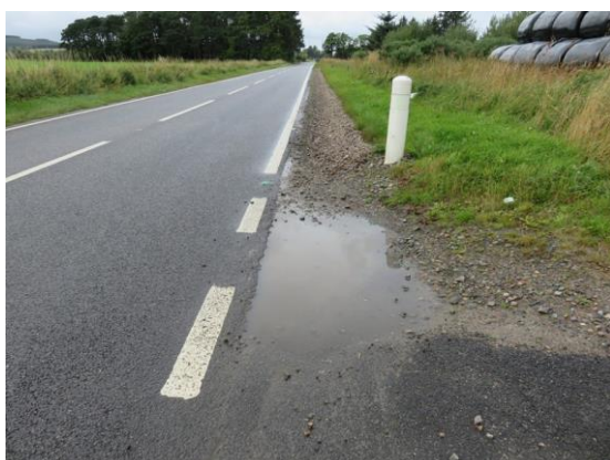
Figure 4.6 Defective drainage (IP29)
