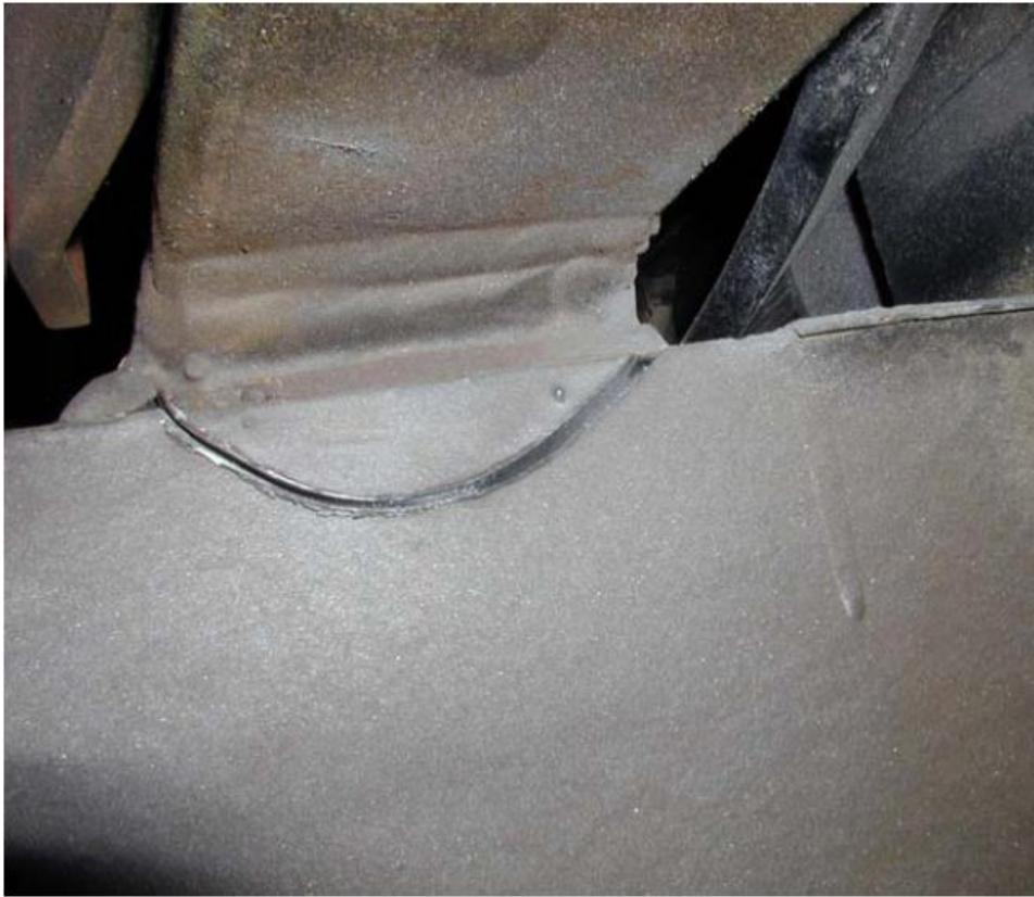
Figure 3 Cable Stayed Bridge (Composite steel-concrete deck) Built 1991 [ Fracture in the support joist immediately below the welded connection to the rail.]
