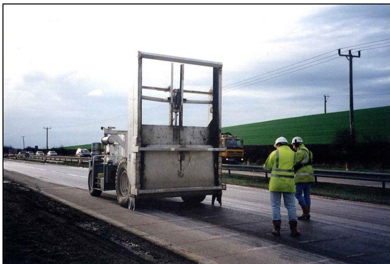
Figure A.1 Standard guillotine breaker used for crack and seat
