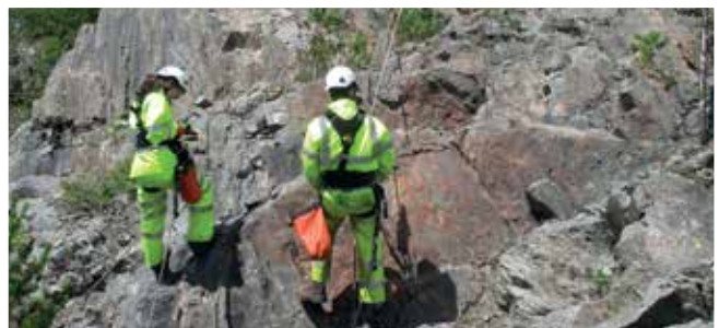
Rope access inspection work
