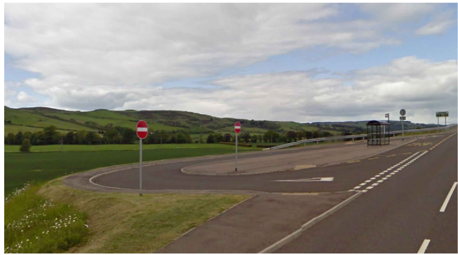
Typical Bus Turning Facility
