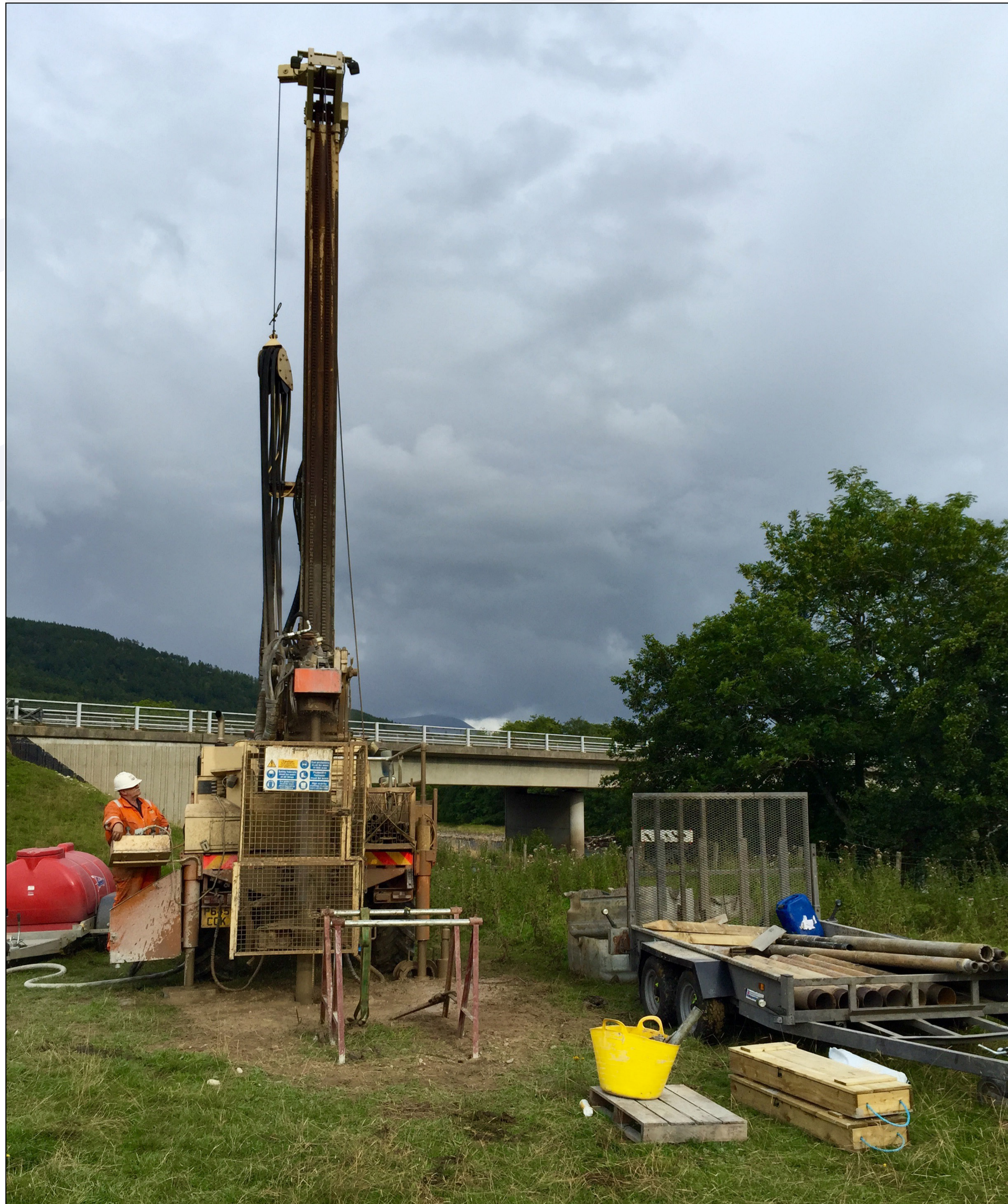
Ground investigation works underway at Pitaldonich Underbridge across the River Garry.
