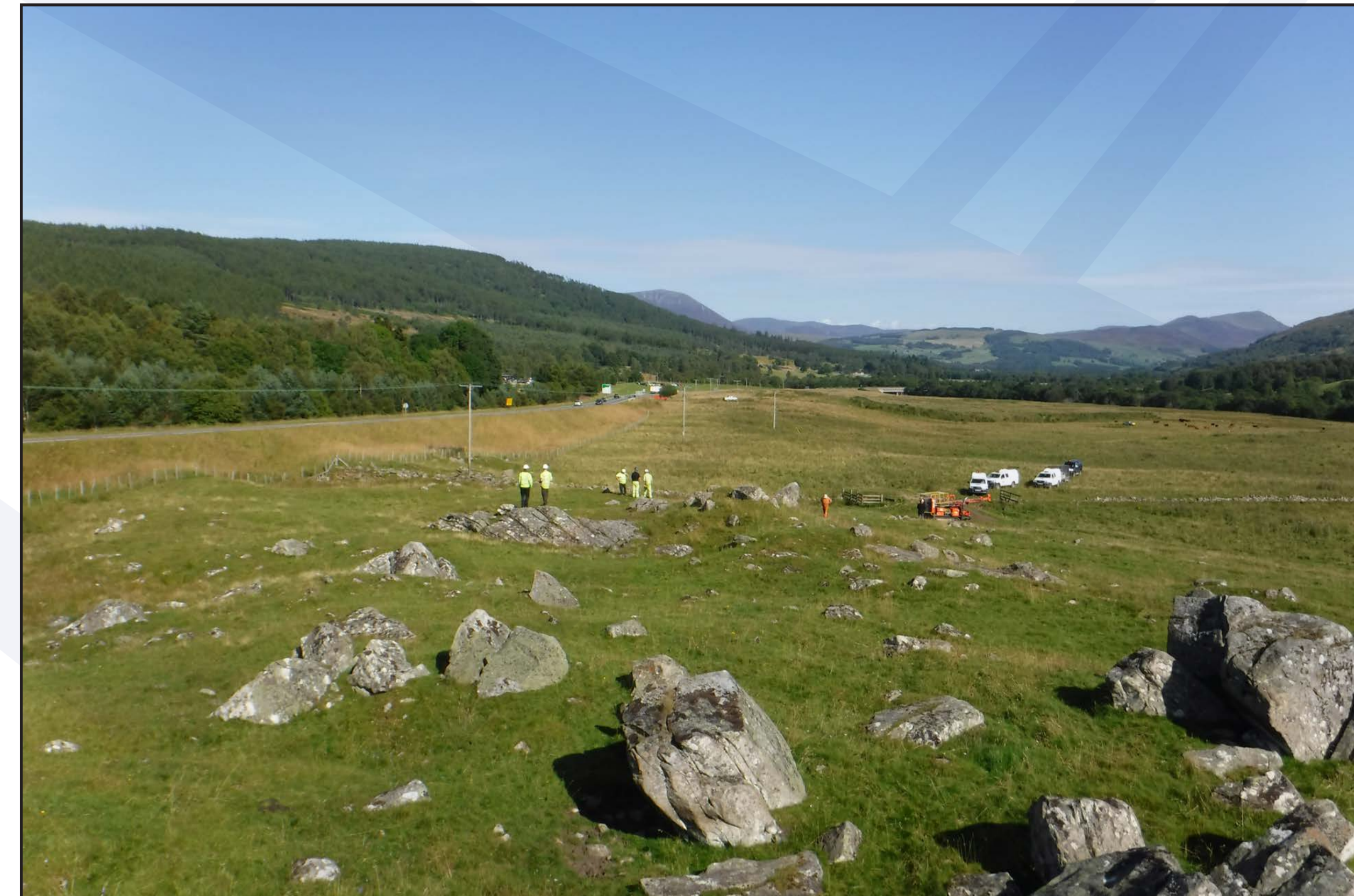
Ground investigation works between Bruar and Calvine.
