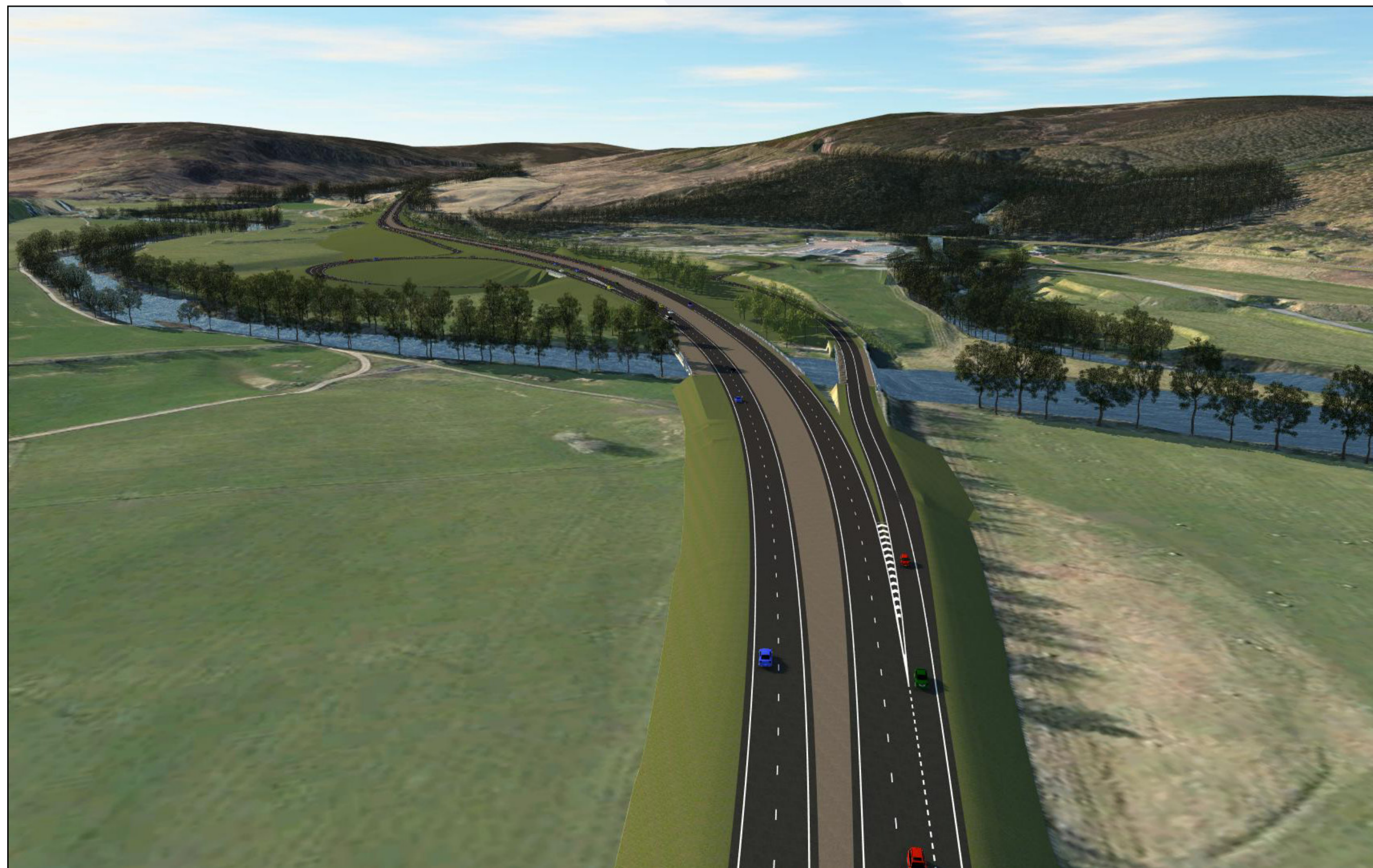
View of the dualled A9 on approach to Pitaldonich Underbridge.
