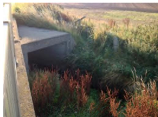
**Diagram 54: Culvert Under the Existing A96 at Auchnacloch (GR - NH 90292 56199 October 2015)**
