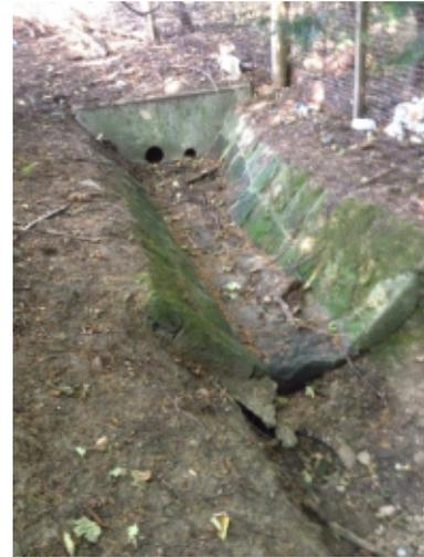
**Diagram 56: Outfall Immediately Downstream of the Existing Auldearn A96 Culvert (Gr - NH 91710 55759 October 2015)**
