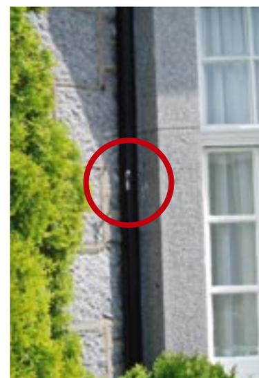
The monitors collect nitrous oxide (NO<sub>2</sub>) from the air, which is an air pollution indicator. Once collected the tubes are sent to a lab for analysis of the levels of NO<sub>2</sub> in the air during that monthly period.
