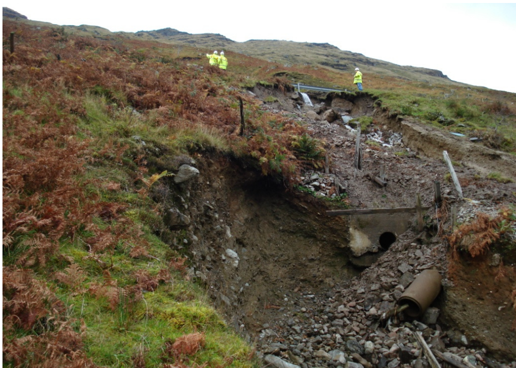
Photograph 6: Culvert discharge pipe
