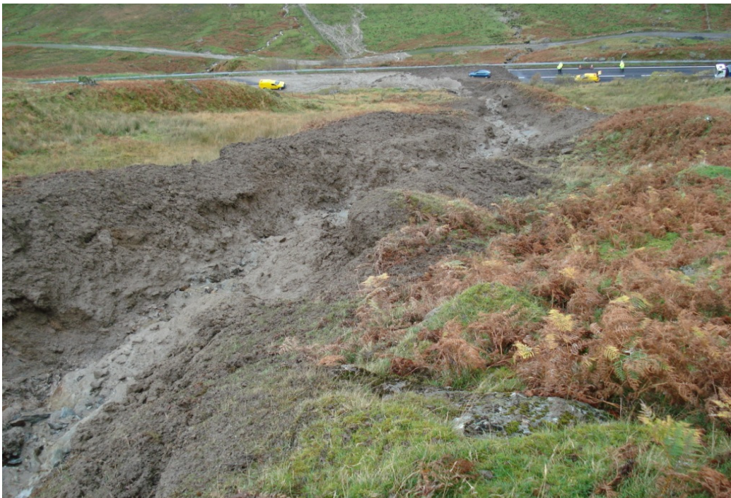
Photograph 4: Debris flow channel looking down slope
