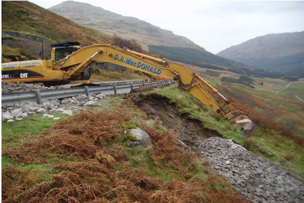
Photograph 13: Construction of buttress fill below the road
