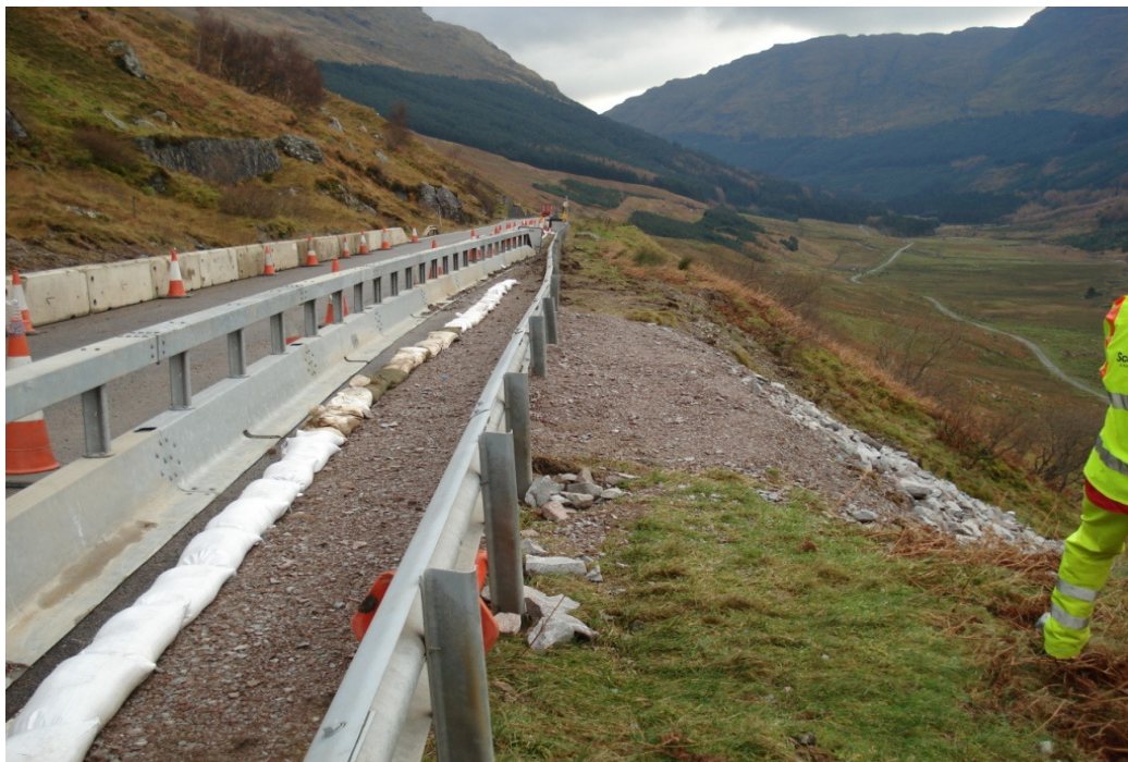
Photograph 14: Granular capping layer on buttress fill adjacent to carriageway
