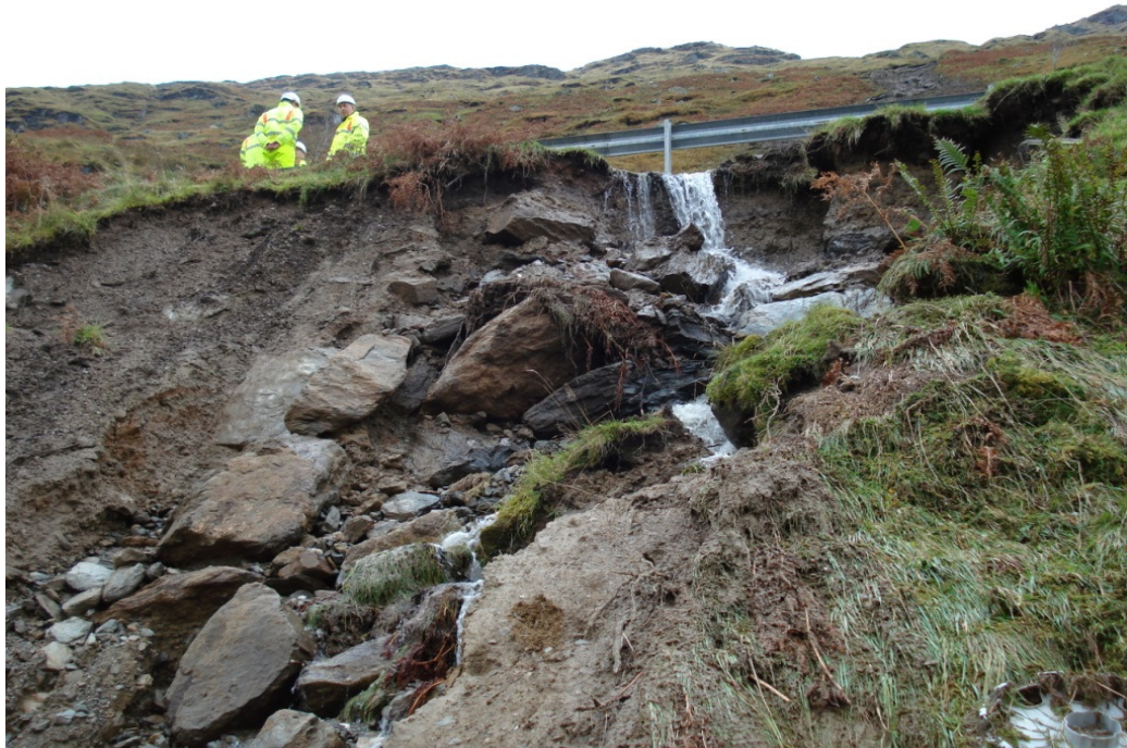
Photograph 5: Erosion channel below the road
