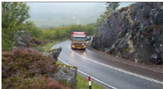
Photo 6 - Some HGV's seen to cross centreline and showing obtrusive rocks.
