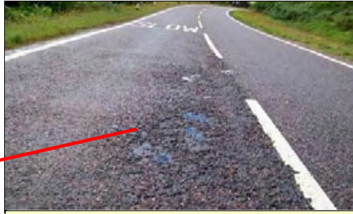
Roughness on CL1 at beginning of bend
