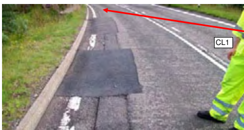
Photo 5: Various patches, some of which have deteriorated, providing an uneven surface of different materials
