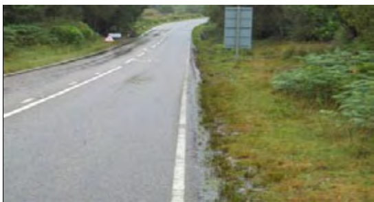
Photo 3 - CL1 - View of edge overrun further down site
