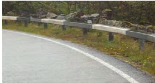
Photo 4 - Evidence of barrier strikes on bend
