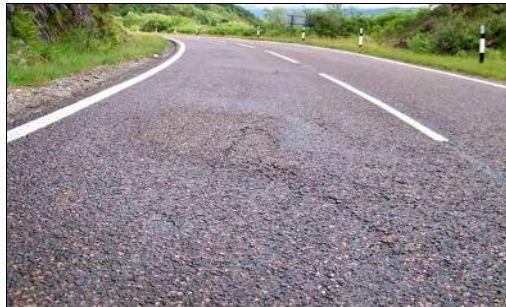
CR1 area of sinking in wheel track
