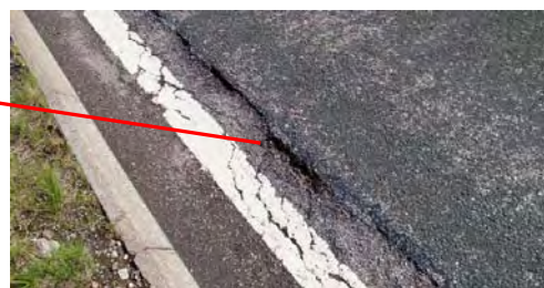
Photo 6: Deterioration of seam on previous repairs on CR1
