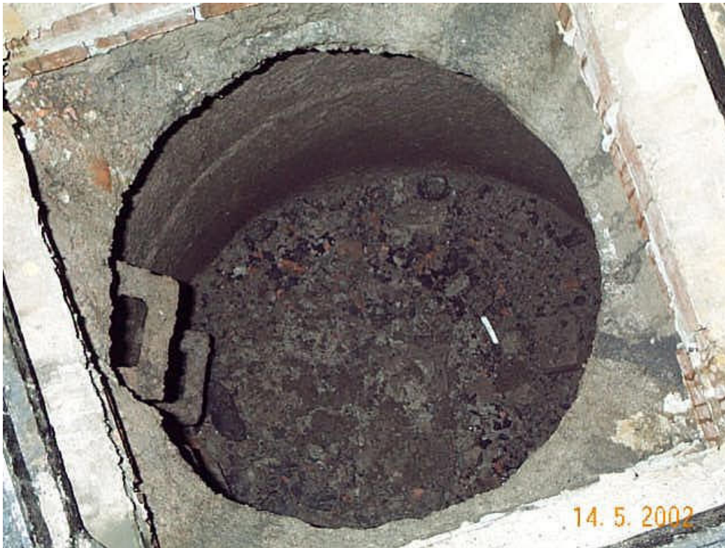
Debris found in manhole E38
