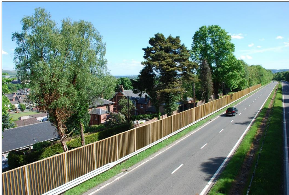
Image 4 – TNAP Noise Barrier installed on M80 at Castlecary
