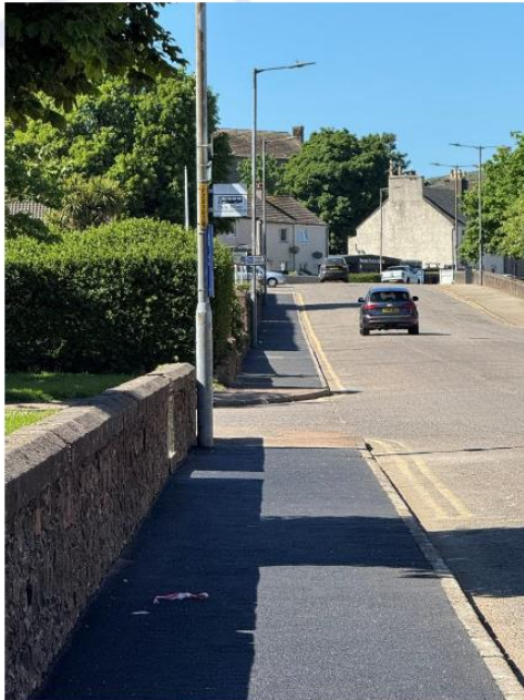
A83 Millknowe Road Campbeltown Footway
