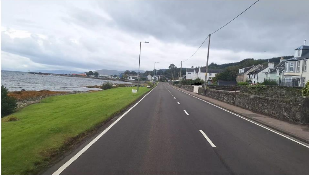
A83 Ardrishaig Surfacing
