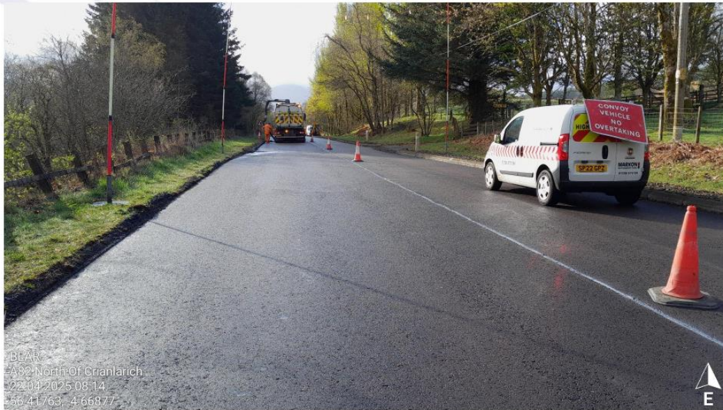
A82 North of Crianlarich Surfacing
