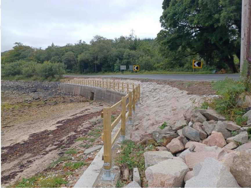
A83 Inveraray Scour Repairs
