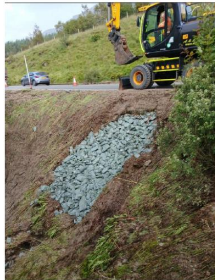
small culvert north of A83 Loch Restil
