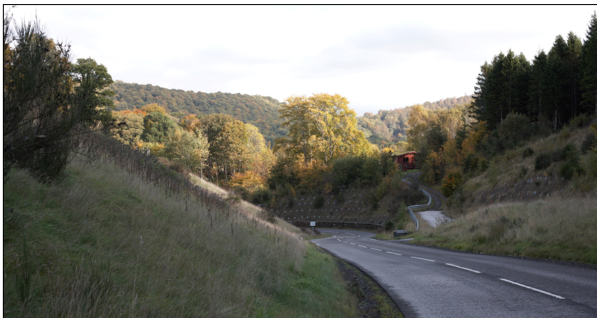
Photograph 11.16: View looking north-east along the A822 (approaching the existing A9)
