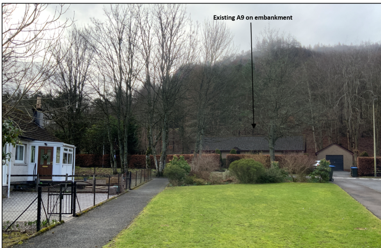
Photograph 11.12: View looking south towards the existing A9 from Carse-na-Tay and 2 Inchewan, Birnam
