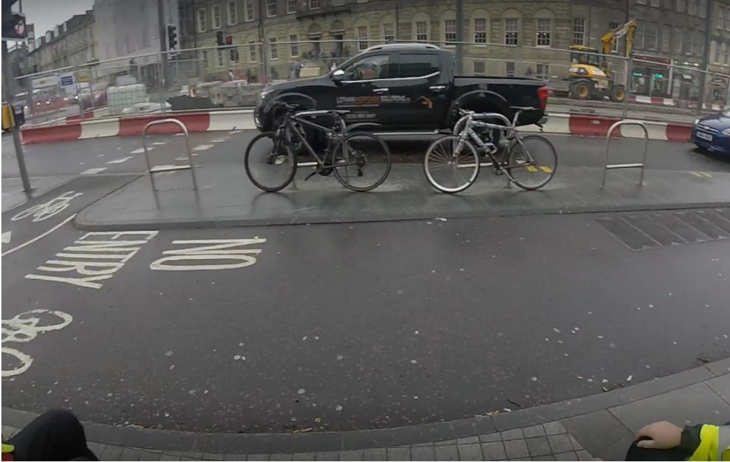
Figure 4-17: Poor contrast between kerb and cycleway surfacing
