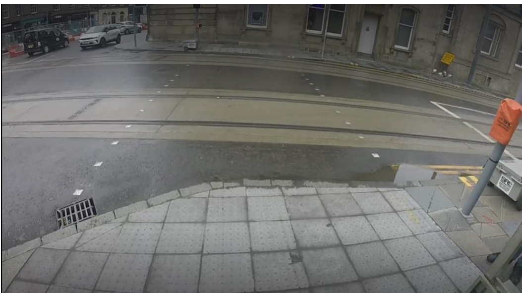
Figure 4-15: Possibility of wheelchair user rolling down graded tactile paving
