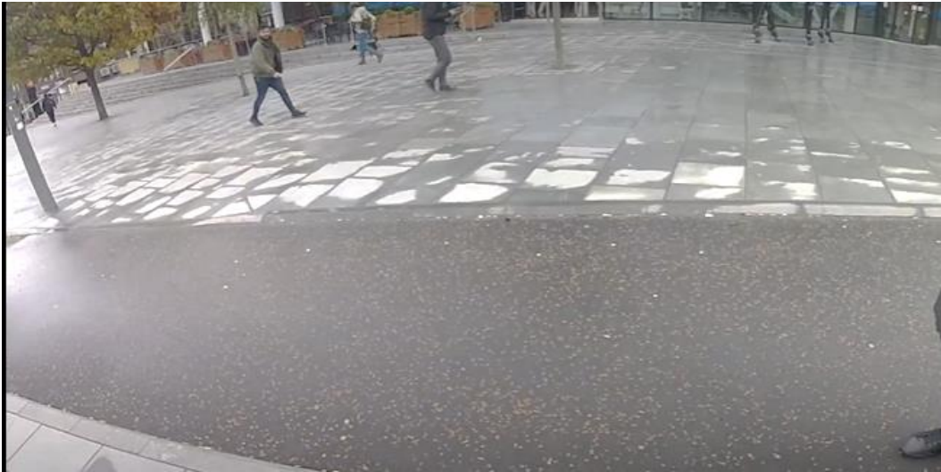
Figure 4-5: Contrast in colour between footway and cycleway
