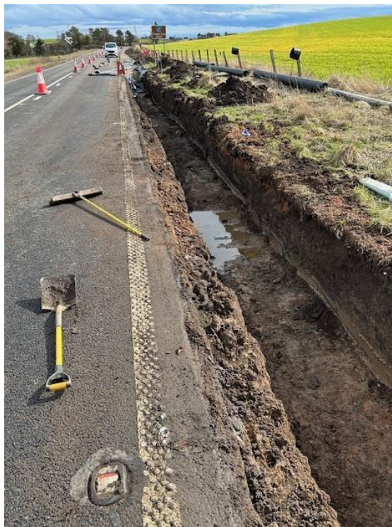
Image 3: Ditches were created after investigations found no formal drainage infrastructure
