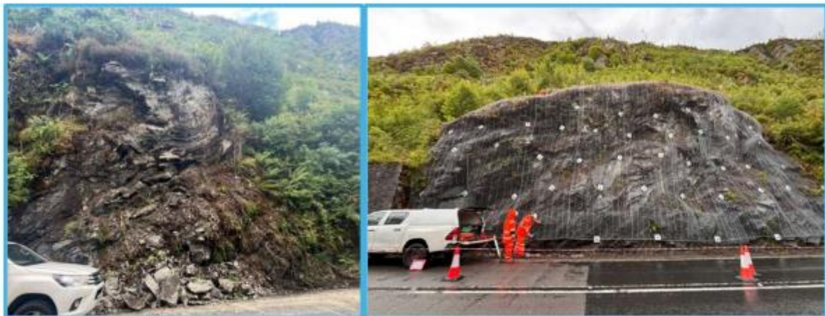
Images 1 & 2: A82 Corran Ferry Rockfall (left) and completed works (right)
