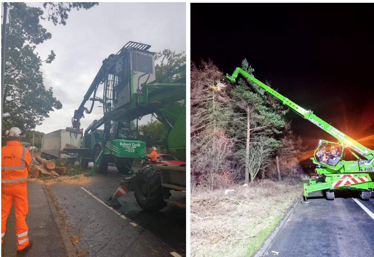
Figure 46 Forestry equipment used on routes to remove diseased trees
