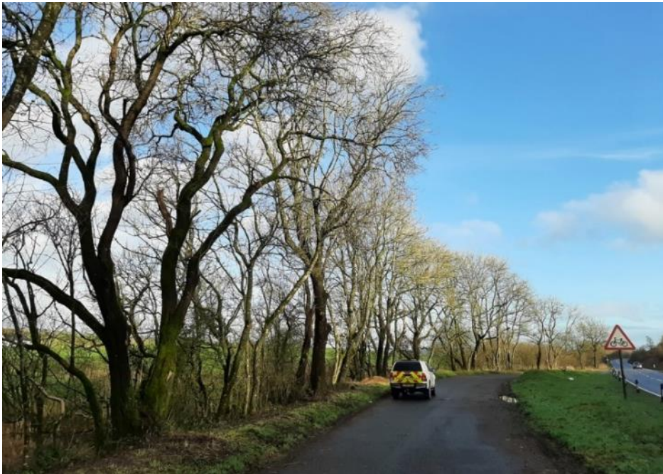
Figure 45 Maturing ash trees affected by ash dieback diseases to the extent that they will need to be felled
