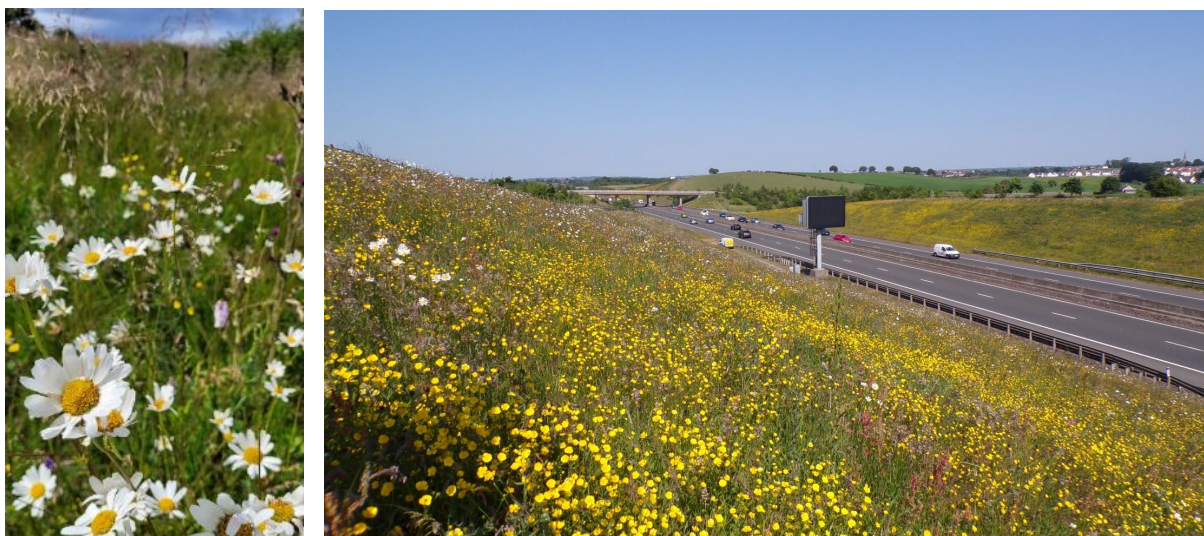
Figure 30 Extensive species-rich seeding and wildflower swards have been successfully established as part of the M80 scheme.
