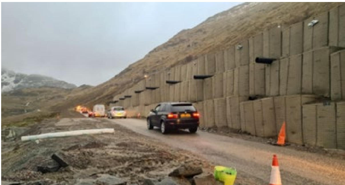
Figure 51 Completed temporary bund from the roadside, OMR
