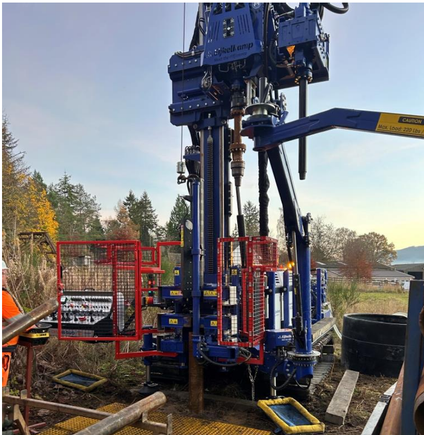
Figure 3. Ground investigation work for A9 Dualling: Tay Crossing to Ballinluig project
