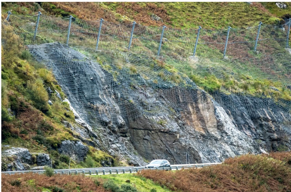
Figure 5. Landslip protection measures on the A83 Rest and Be Thankful
