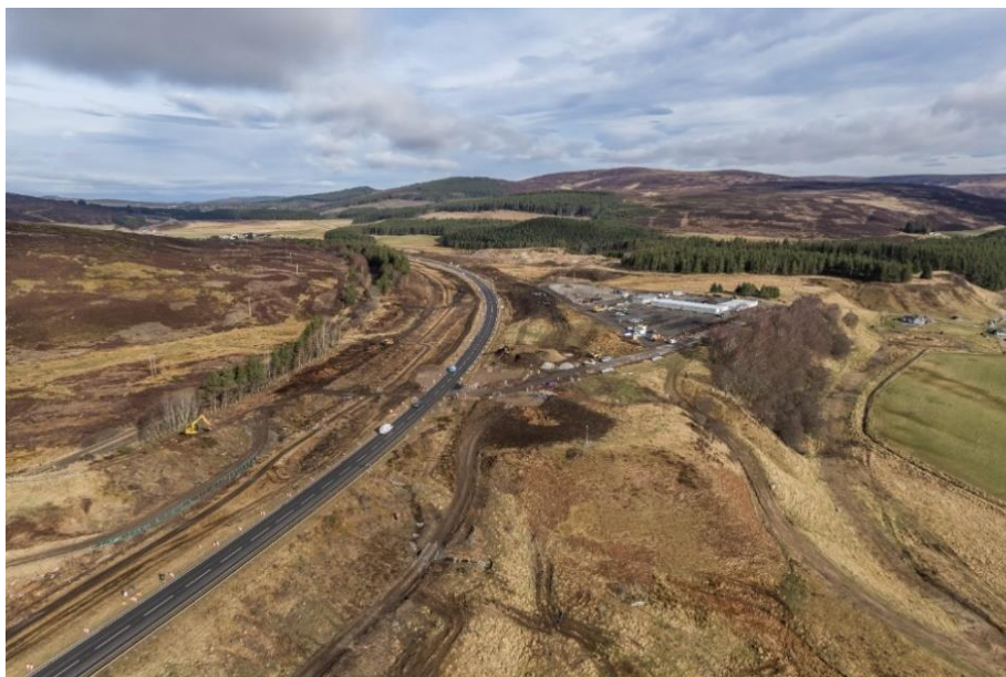
Figure 2. A9 Dualling: Tomatin to Moy project site compound under construction
