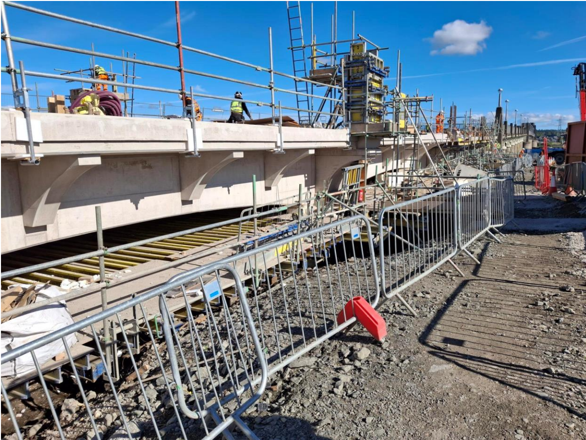
Figure 9. The A985 Kincardine bridge southern piled viaduct replacement
