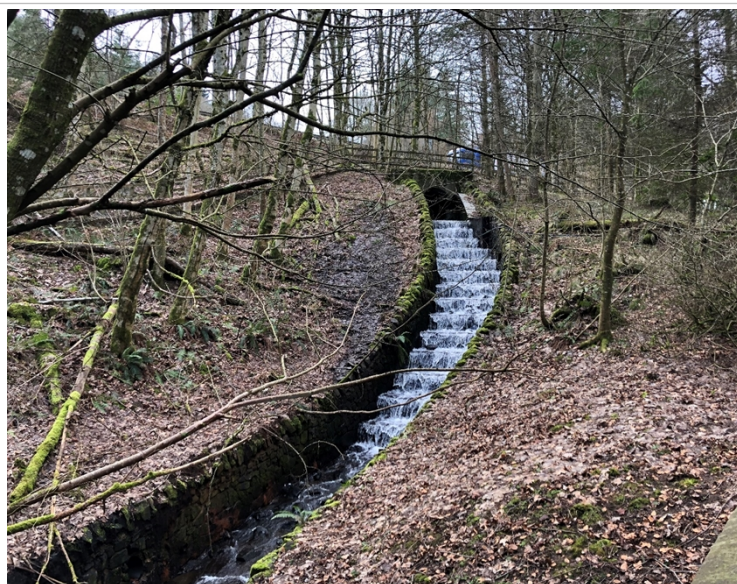
Photograph 1: WF1 Existing A9 culvert outlet and downstream cascade
