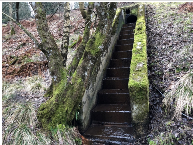
Photograph 3: WF2 Existing A9 culvert outlet and downstream channel
