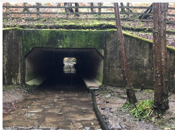
Photograph 21: WF12 (Mill Lade) Existing A9 Culvert outlet and downstream channel
