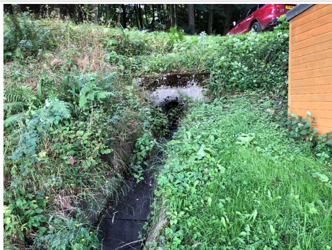
Photograph 11: WF05A Existing Access Track culvert outlet and downstream channel
