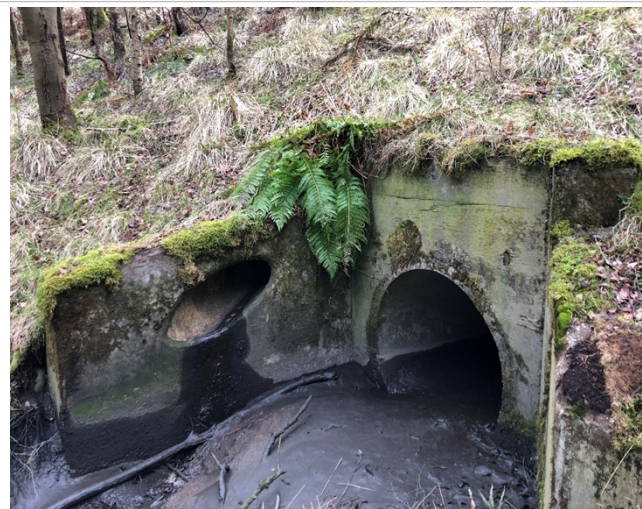
Photograph 9: WF05A Existing A9 outlet and downstream channel
