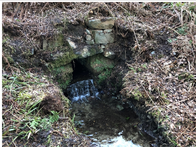
Photograph 5: WF05 Existing A9 culvert outlet and downstream channel
