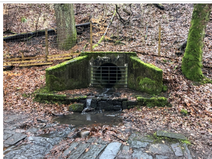
Photograph 21: WF12 (Mill Lade) Existing A9 Culvert outlet and downstream channel
