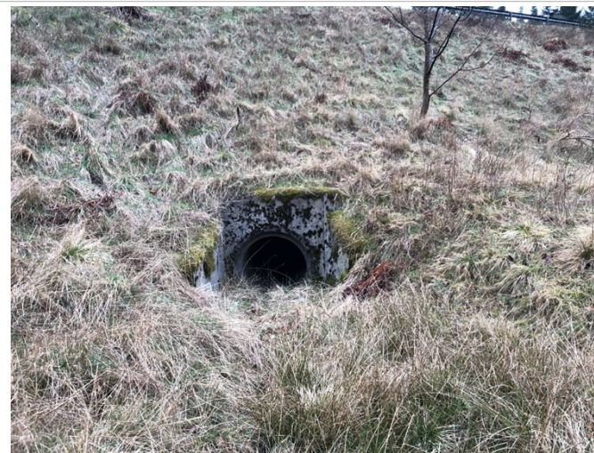
Photograph 10: WF05A Existing A9 culvert inlet and upstream channel
