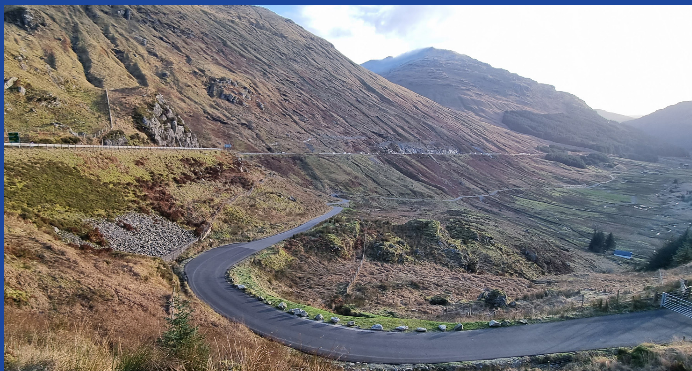
Northern end of the Old Military Road
