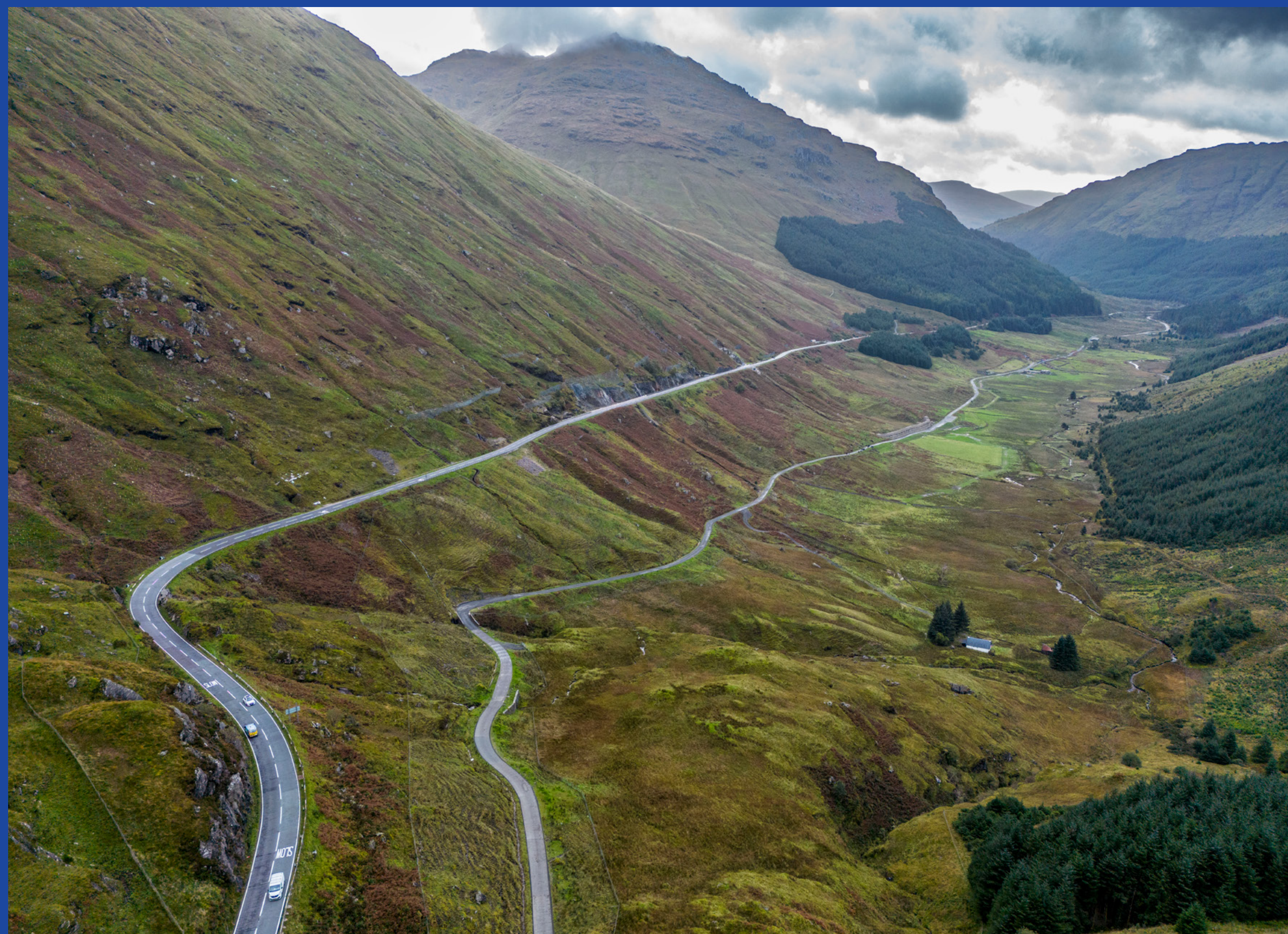
Aerial image of A83 and Old Military Road looking south east
