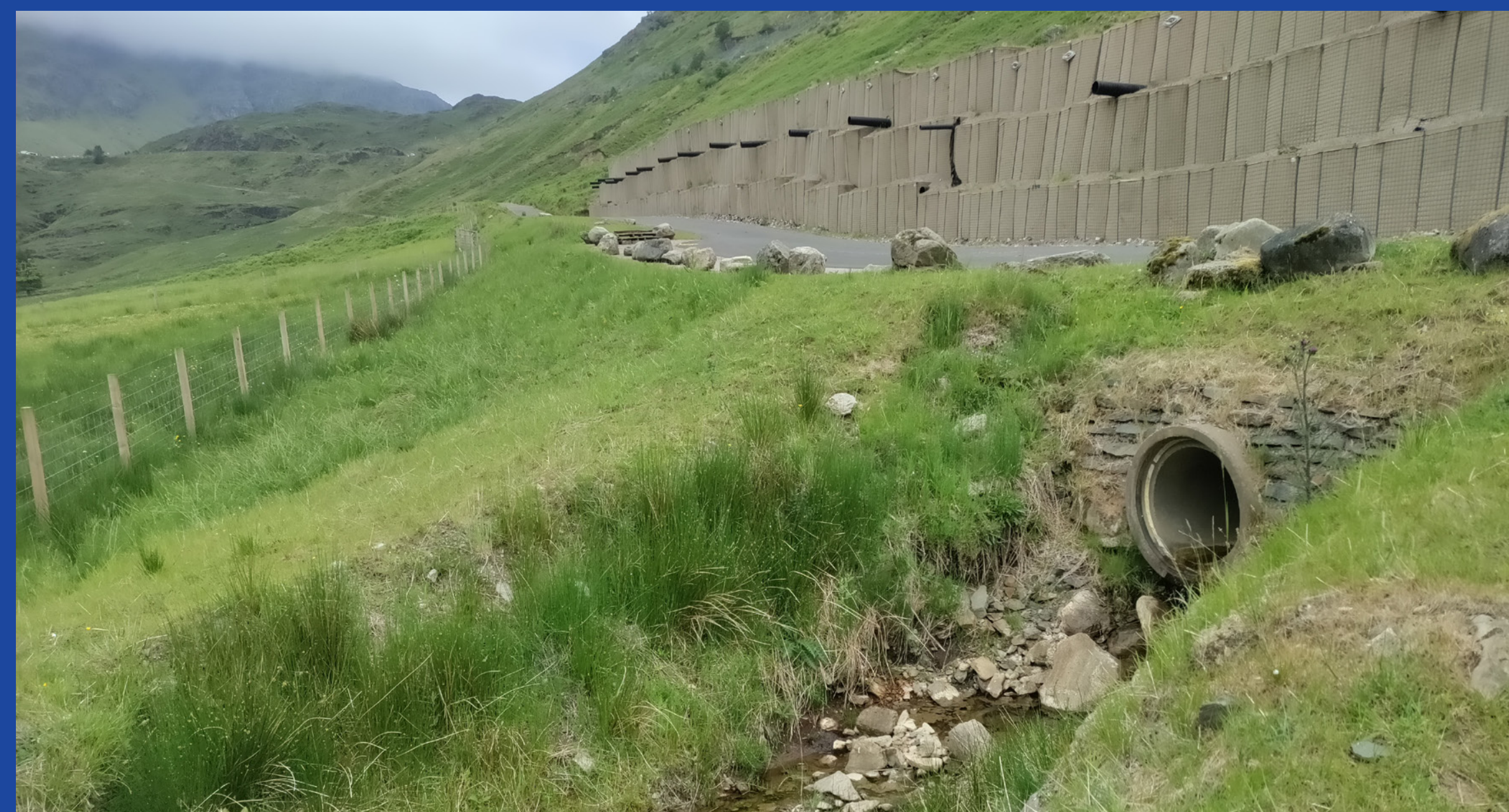
Hesco bund on the Old Military Road
