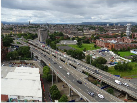
Aerial picture of the M8 Woodside Viaduct
