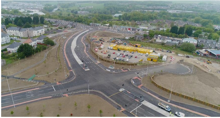
The A92/A96 Haudagain Improvement scheme during construction
