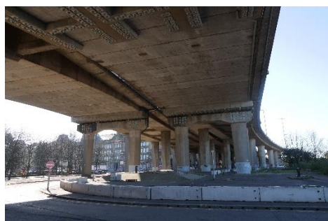
The M8 Kingston Bridge works
